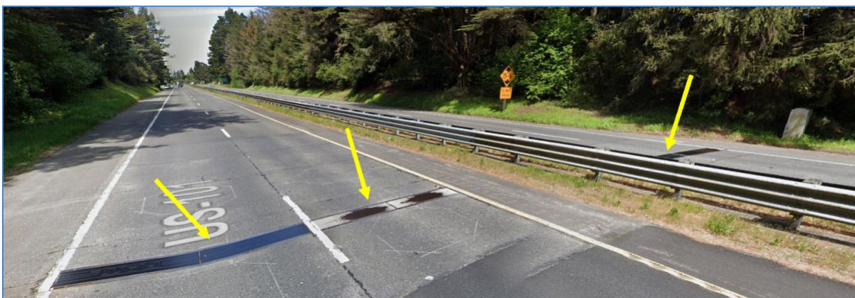
Figure 37. Weigh-in-Motion Station at Loleta on US-101
