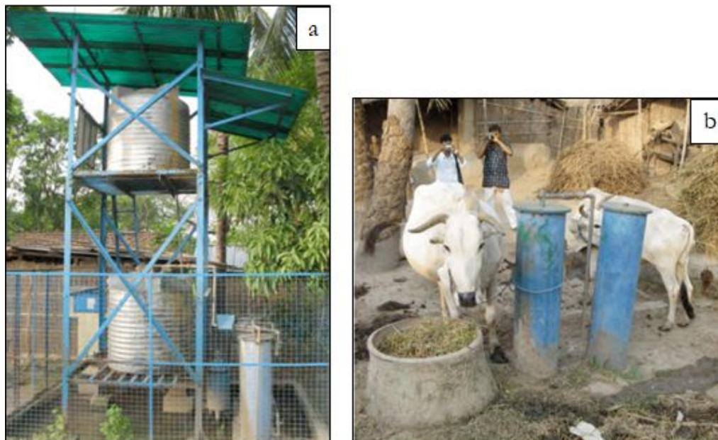
**Fig. 5.1** Photographs of arsenic treatment devices in Murshidabad District of West Bengal, India. Panel a), Working arsenic filter, (typical for 5% of installed units at 1-year after installation). And, Panel b), Defunct arsenic treatment unit, (typical of 95% of units at 1-year after installation)
