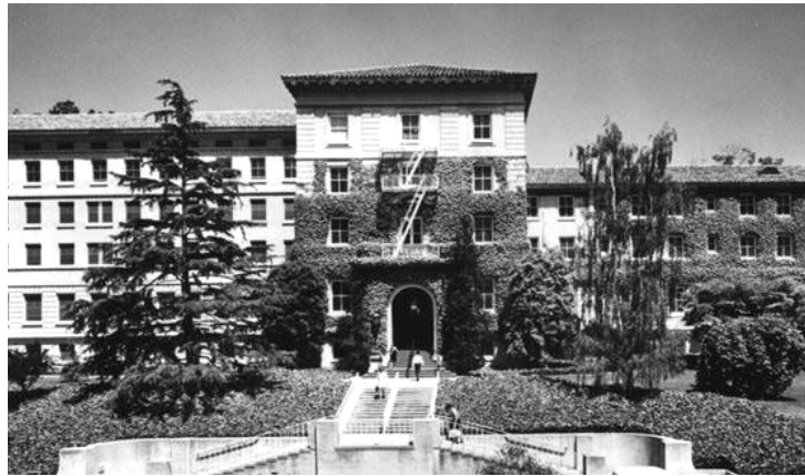
Ernest V. Cowell Memorial Hospital at 2215 College Ave. Berkeley, CA before its demolition in 1993. The building later became eligible for the National Register of Historic Places and considered a landmark of social history. Credit: National Park Service.
