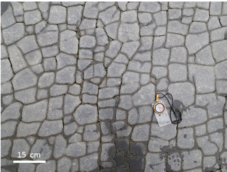
Fig. 4. (a) Bedding plane joint pattern from Lower Jurassic limestone of north Somerset at (a) Lilstock and (b) Blue Ben. In both examples the bedding planes are subhorizontal and the joints are subvertical and confined to the limestone unit.
