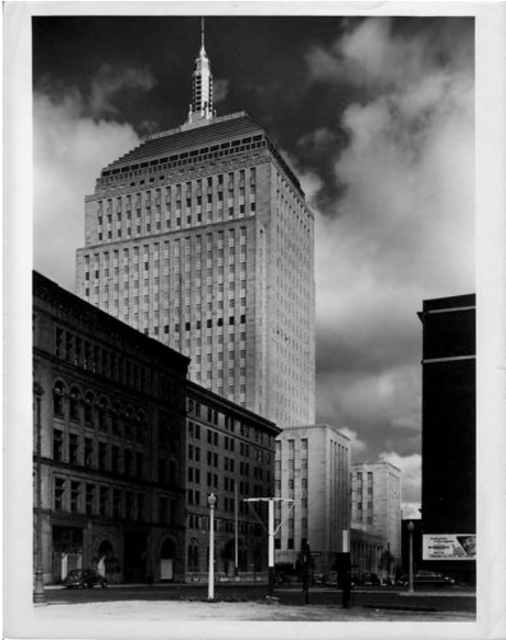
Figure 2.6. A stunning photograph of the John Hancock Insurance Company tower in Boston, probably taken not long after it was completed in 1947. The design is by Cram & Ferguson. Source: Boston Public Library, Fine Arts Department, John Hancock Insurance Company Collection.
