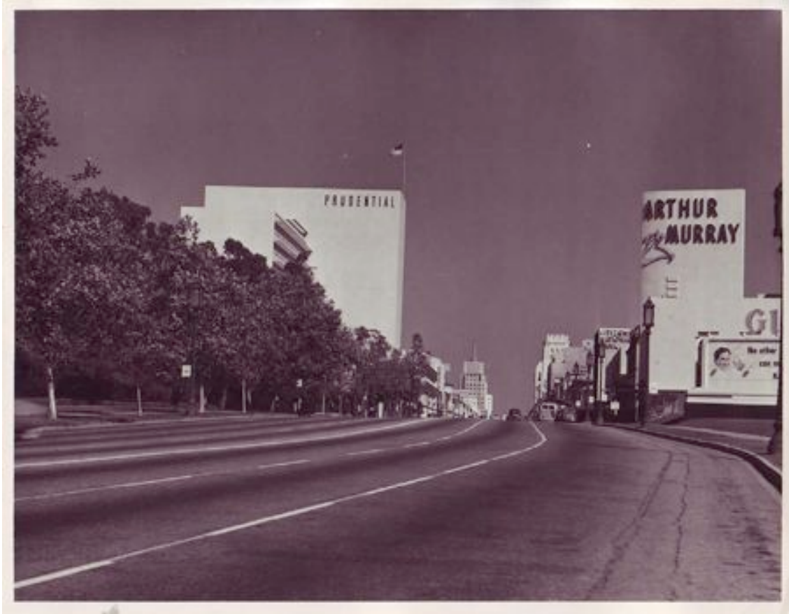
Figure 1.6. A view of the Western Home Office driving east on Wilshire Boulevard, ca. 1950. Wurdemann & Beckett used the mechanical core of the building to design a billboard. Source: PA 17–57.
