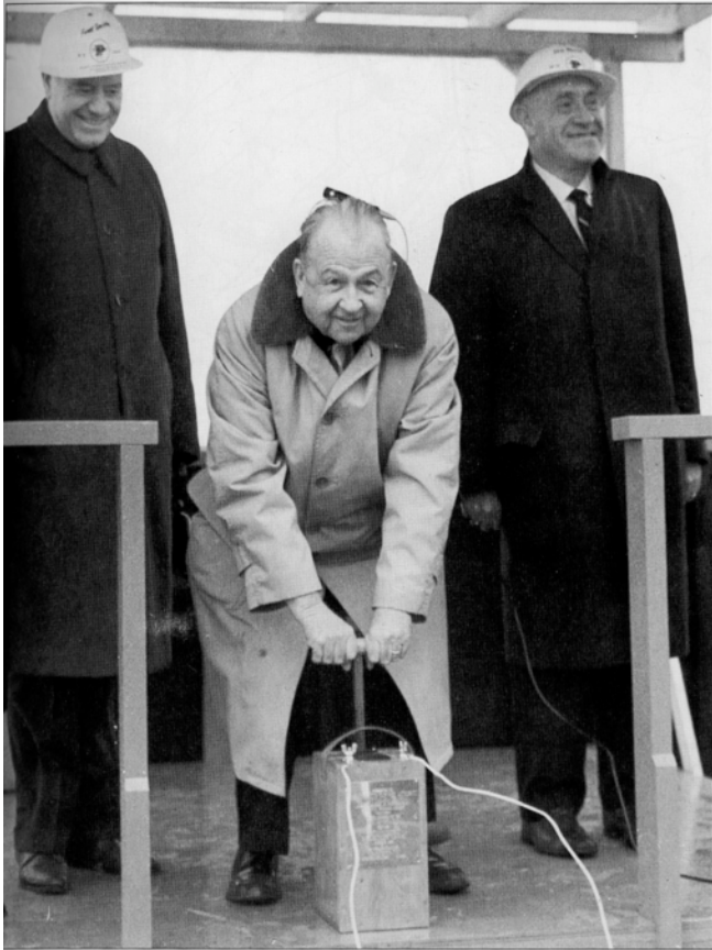
Figure 4.4: William F. Callahan depresses the plunger that inaugurated the Mass Pike Boston Extension construction project. On his left is Lou Perini, the contractor. On his right is Fred Smith, Prudential's main negotiator in Boston. Source: Perini Corporation, Framingham, Massachusetts.
