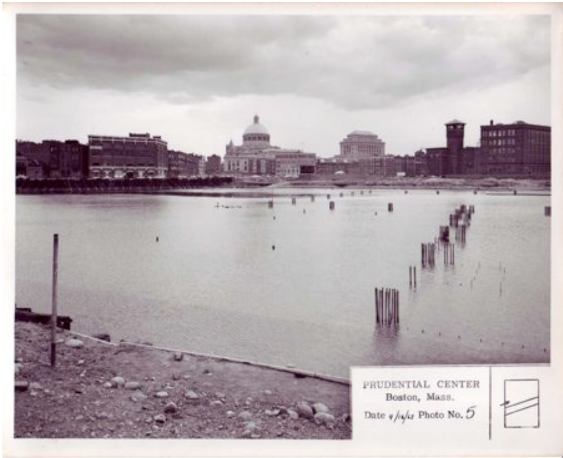
Figure 5.18. When Prudential ordered that the de-watering pumps be shut-down in 1960, the Prudential Center site was flooded, as shown in this 1962 photo. Source: Perini Corporation Archives.
