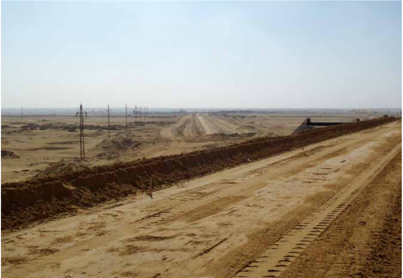
Figure 7.3. North of L Basin showing recent destruction as of December 2014.
