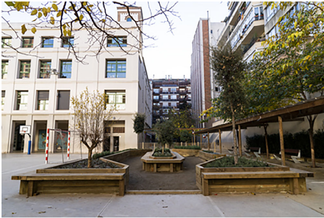
FIGURE 1 A schoolyard transformed into a climate shelter in Barcelona. Interventions include a new garden with drought-tolerant trees and herbs, unsealed pavement, a gazebo with a vine, water points and seating arrangements. Source: Ajuntament de Barcelona.
