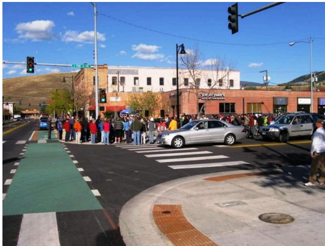
Figure 4.16: Bike lane painted pavement through an intersection
