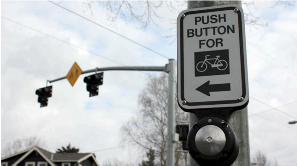
Figure 4.9: High-intensity activated crosswalk beacon adapted for bicycle use
