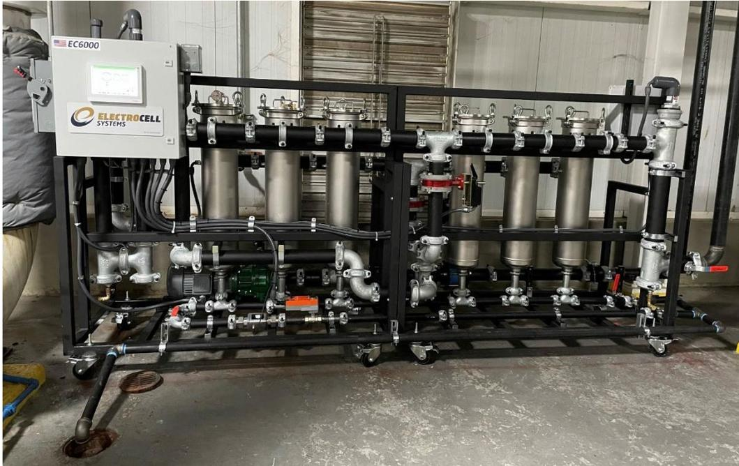
Figure 2. ElectroCell Systems Model EC-6000 installed at Nissan Canton
