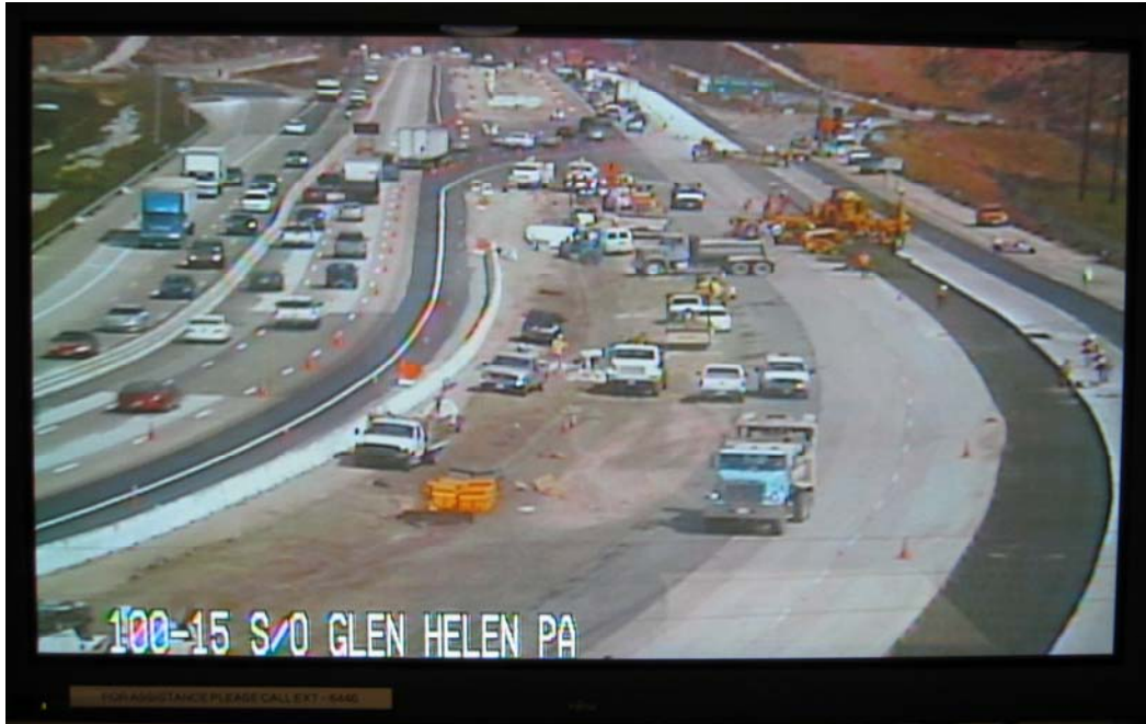
Figure 5: Monitoring of construction and traffic in the project command center.
