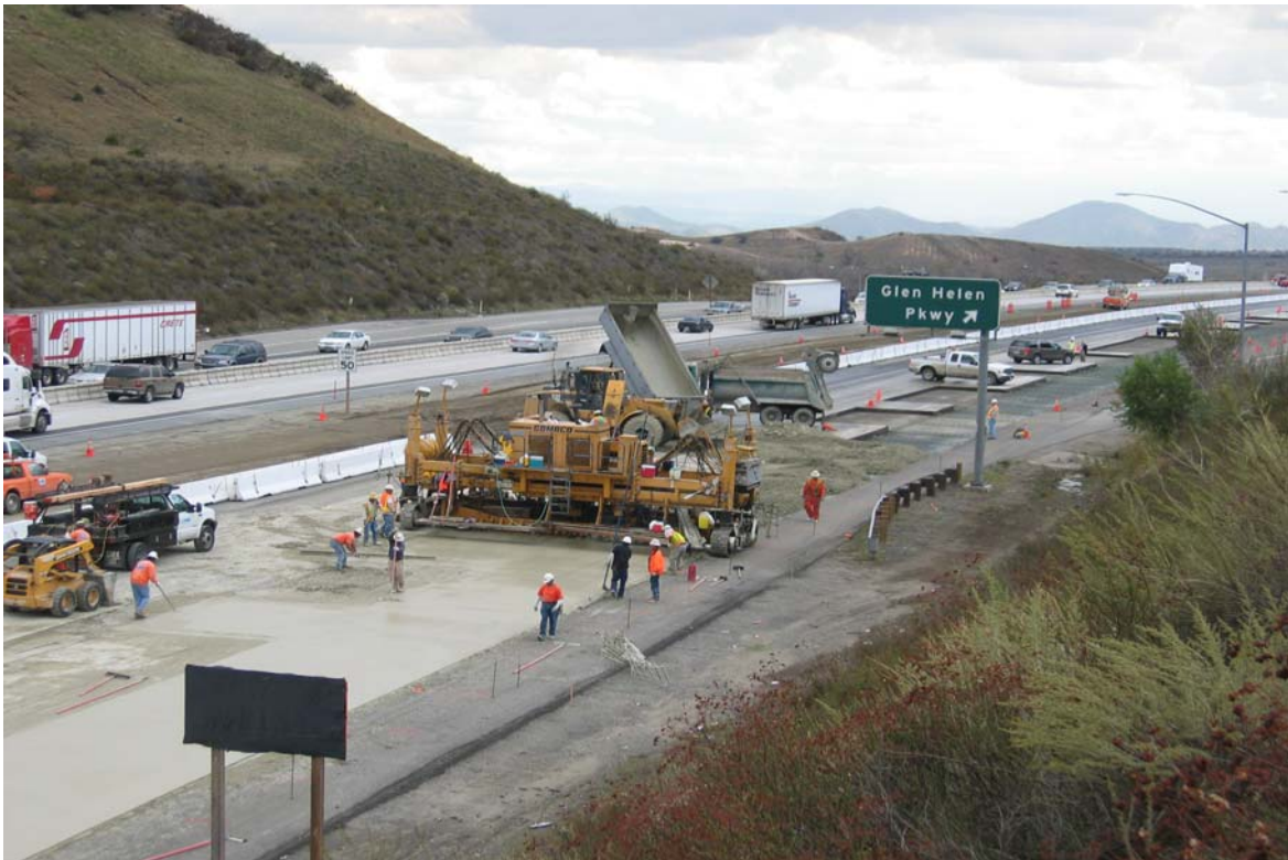
Figure 8: Construction and traffic operation during I-15 Devore reconstruction.
