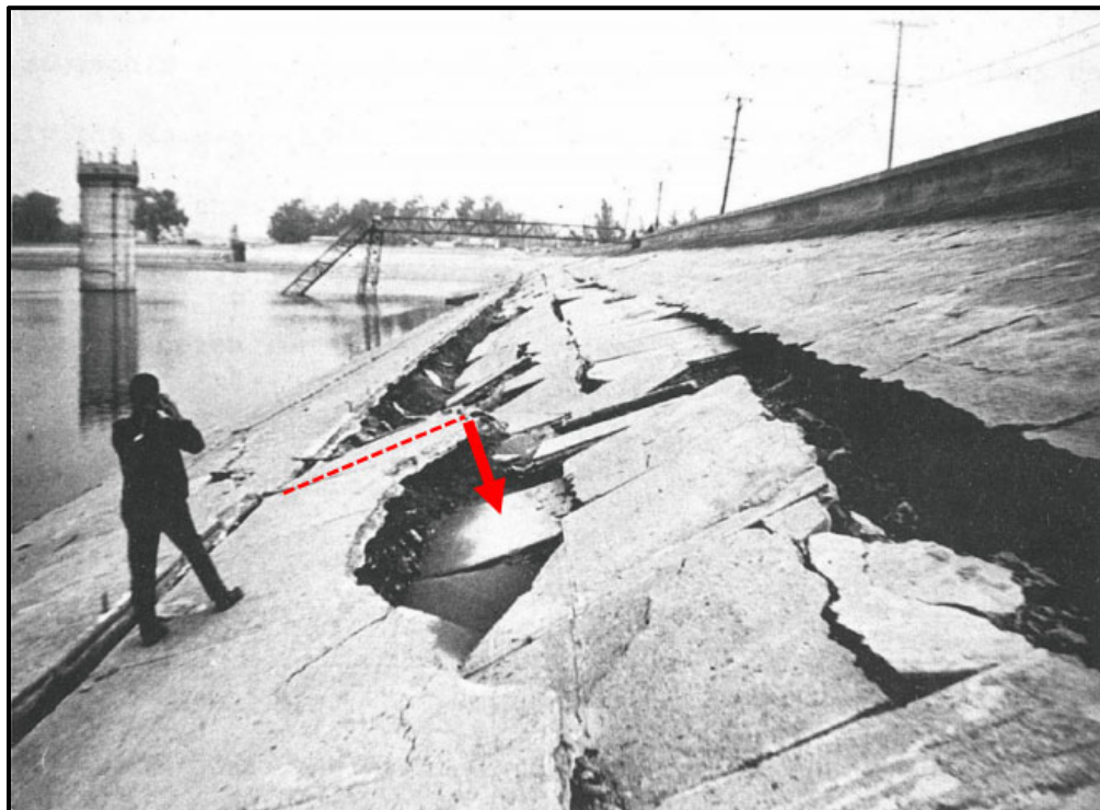
Figure 5-3: Slide scarp on upstream face of the USFD after the 1971 San Fernando earthquake (Seed et al. 1973)
