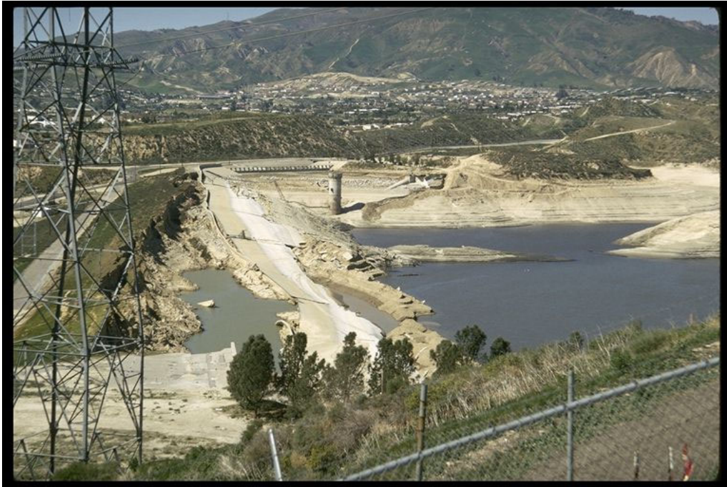
Figure 4-2: The Lower San Fernando Dam after the 1971 San Fernando earthquake (looking West) showing conditions after reservoir drawdown. [Steinbrugge Collection, 1971; NICEE Library, U.C. Berkeley]
