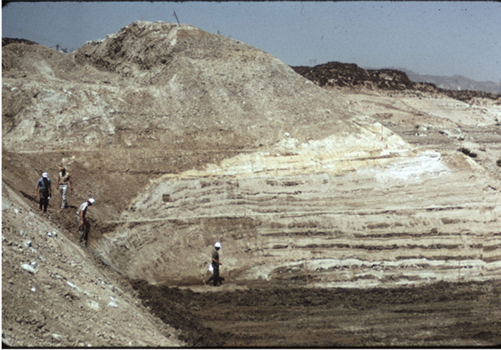
Figure 4-7: Photograph of the side wall of a post-earthquake excavation through the upstream hydraulic fill showing distinct layering within the hydraulic fill zone. (H.B. Seed personal collection)
