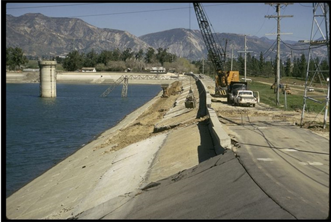
Figure 5-2: Repair of damage to the crest and upstream concrete facing of the Upper San Fernando Dam after the 1971 San Fernando earthquake (Steinbrugge Collection, NICEE library, U.C. Berkeley)
