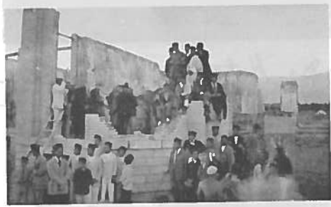
Laying Cornerstone Sept-1924
