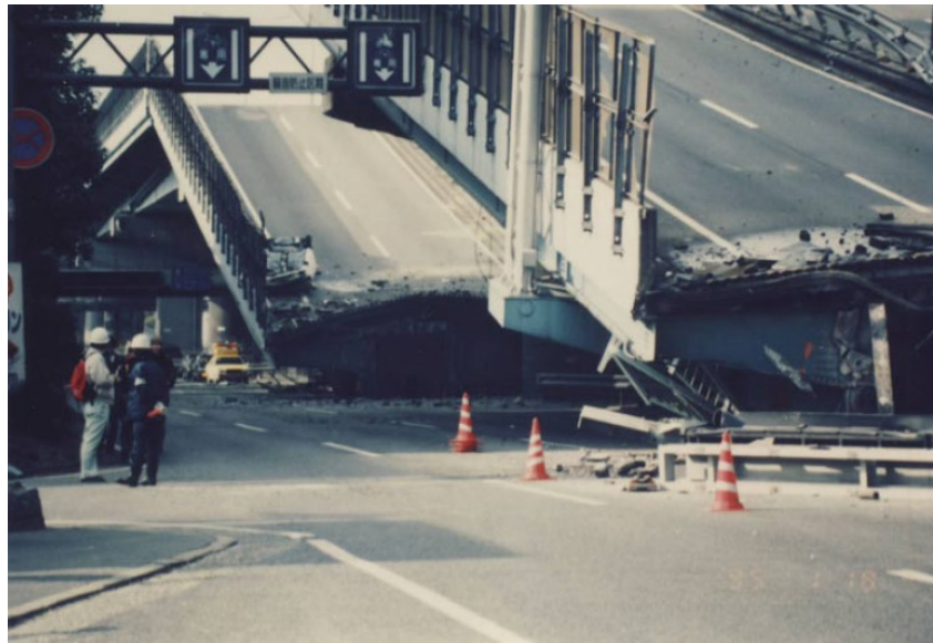
Figure 2.4. Collapsed bridge segment where pounding was a contributing factor (1995 Kobe earthquake).
