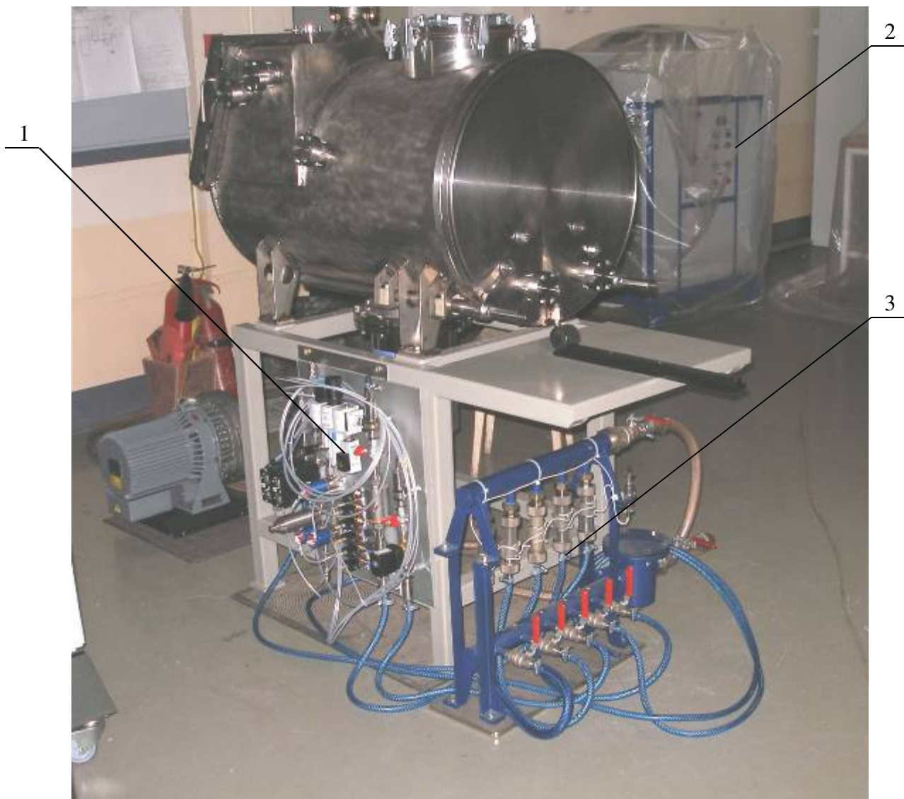
1 – Tamiris 400-f media-panel; 2 – water cooler BTXO-8-C-IIB(M); 3 – water collector-distributor
