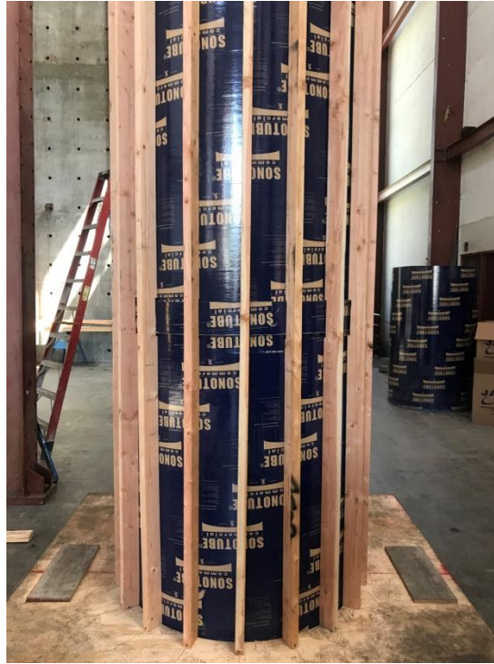
Figure 2–14: The Sonotube® used as formwork for the column (Lotfizadeh, 2019).
