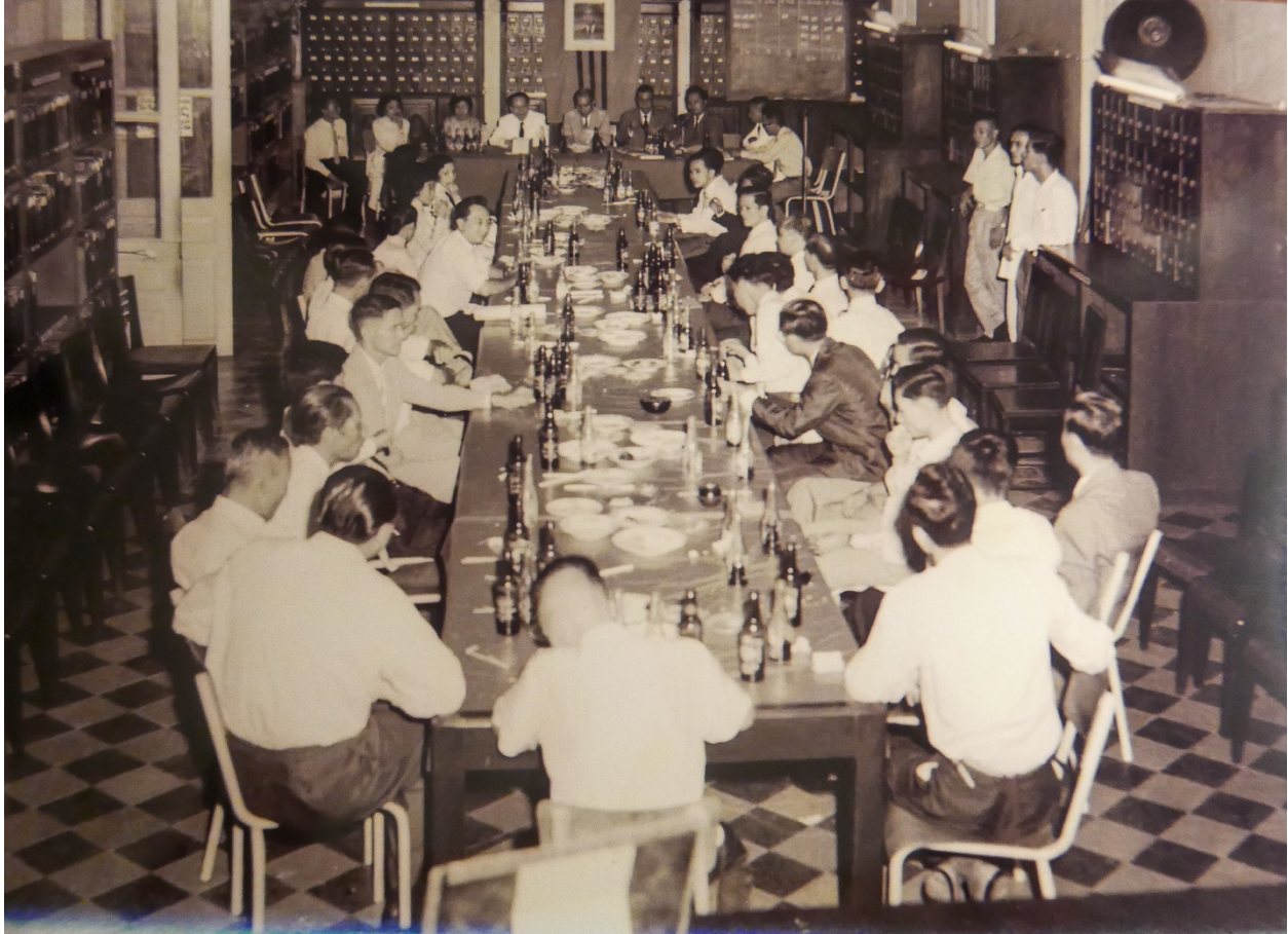
Image 5-9 Bricklaying celebration on April 3, 1956 in the existing National Library building at 34 Gia Long. For additional photographs, see Appendix C.
