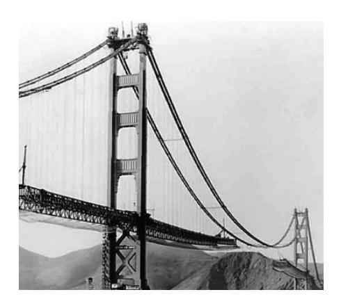
Golden Gate Bridge deck hung from cables while under construction. photographic print: b&w.  $20 \times 21 \text{ cm}$ . (7 3/4 x 8 1/4 in.) 1965
