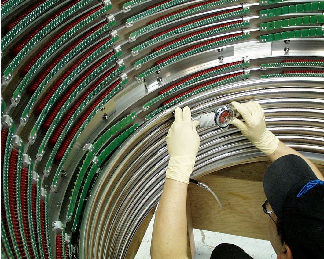
Figure 2.3 View of the inside of the column during assembly showing the resistor and MOV chains.
