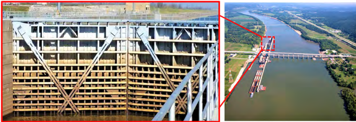
Figure 1: Greenup locks and miter gate
