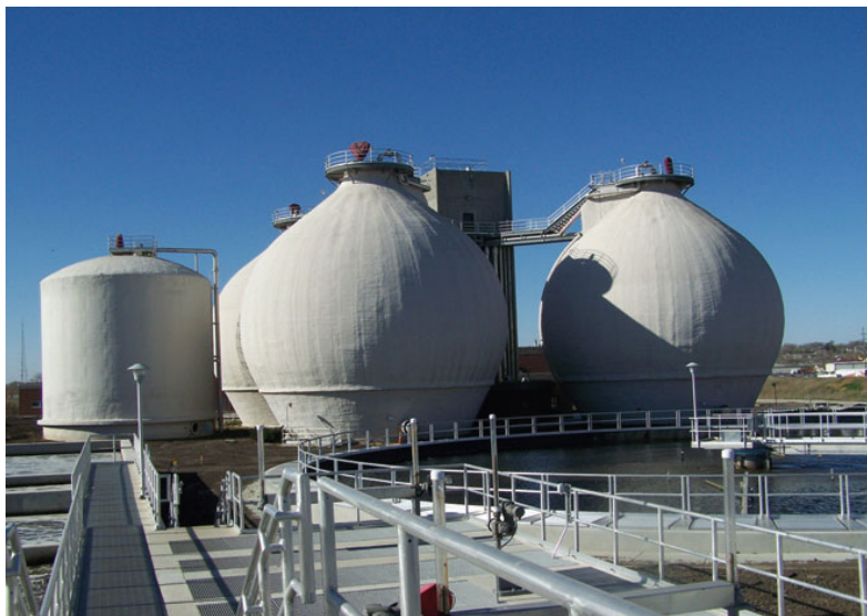
Figure 38. Anaerobic digesters at a wastewater treatment facility
