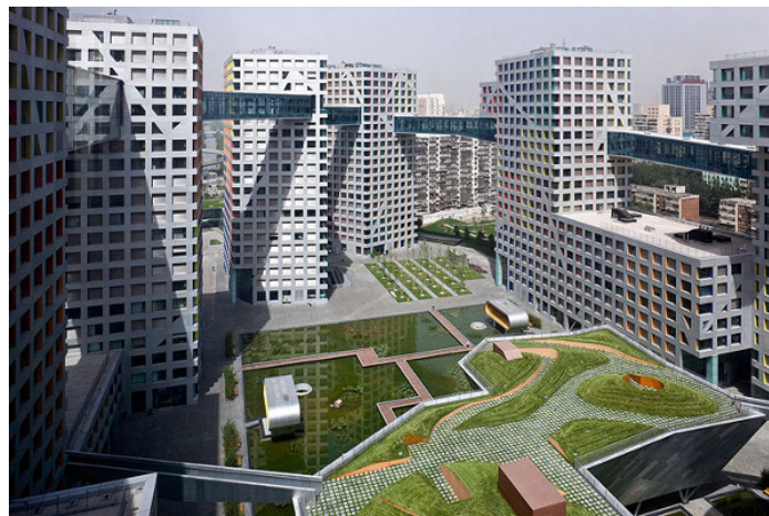
Figure 12. Beijing's linked hybrid at Dongzhimen meets two-thirds of heating/cooling demand with GSHP technology
