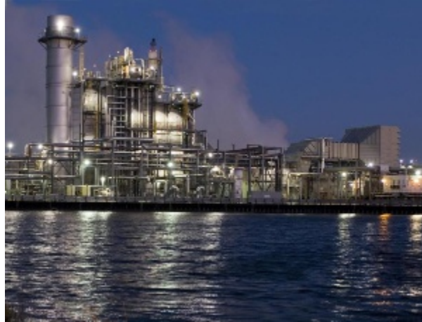
Figure 19 ExxonMobil's Beaumont Refinery in Beaumont, Texas operates a 470-megawatt CHP system that achieves an operating efficiency of 88%
