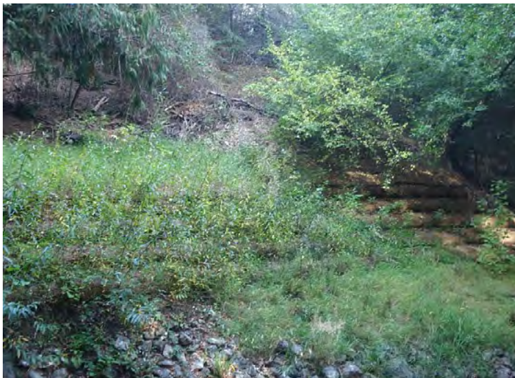
Figure 22 Successful willow planting in sunnier conditions compared to shaded willow live pole planting that did not survive.
