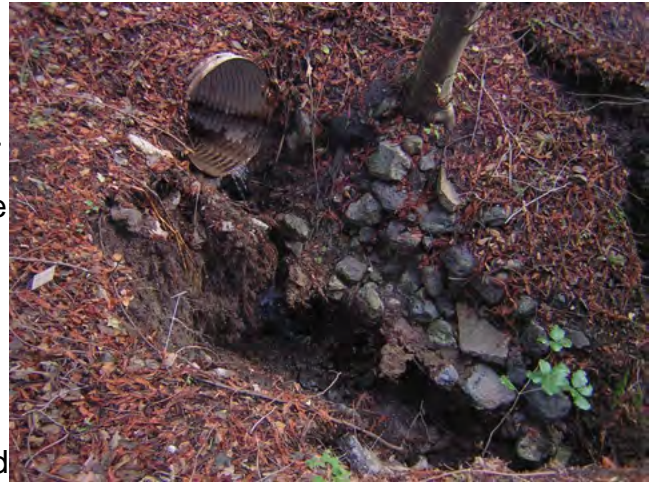
Figure 1. Culvert on Winter Creek in 2005.
