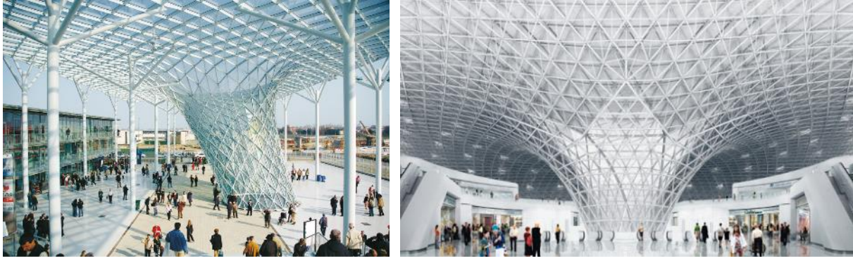
Figure 5-26. Examples of funnel/torus like structures for large continuous roof canopies. Left: New Milano Trade Fair Rho-Phero. Image from: Studio Fuksas (2005). Right: New Mexico City Airport. Image from: Foster and Partners (2014).
