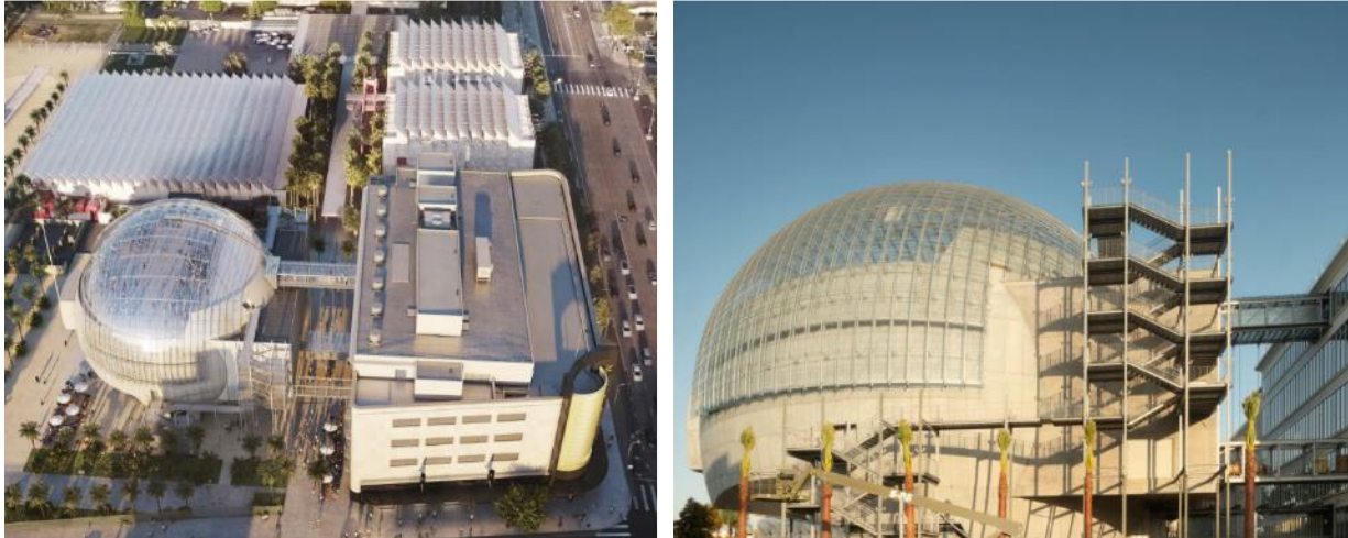
Figure 5-33. The glass dome of the Academy Museum of Motion Pictures by RPBW (2019). This built example and location motivate the experiment conducted in this section. Images adapted from: RPBW (2019).
