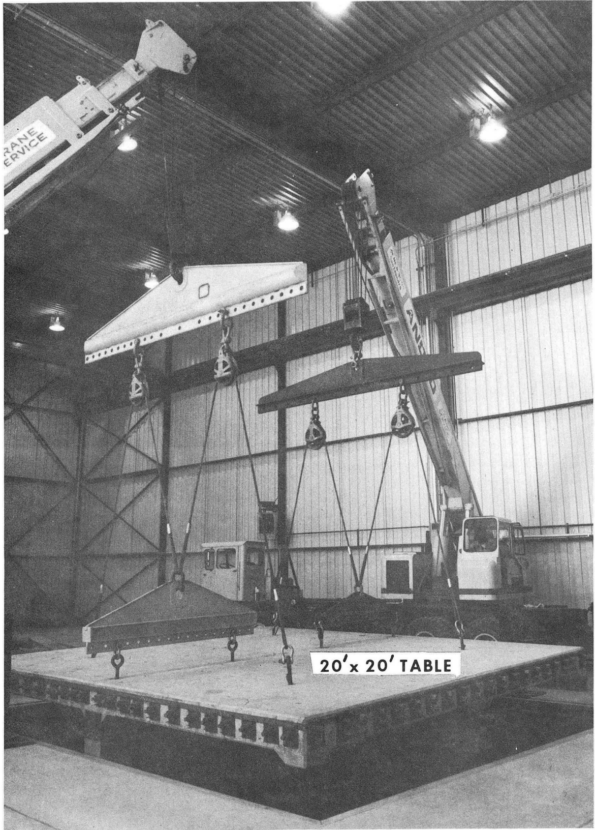
FIG. 3-1. 20 X 20 FOOT PRESTRESSED CONCRETE TABLE BEING LOWERED IN PLACE.
