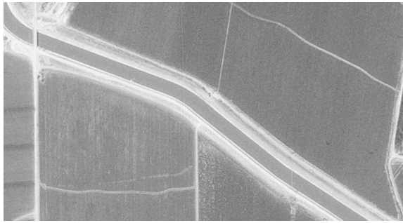
Fig. 19. Canal at the Crowslanding facility.
