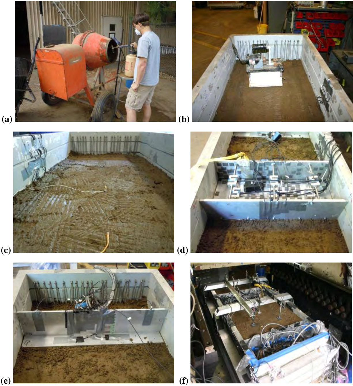
Figure 3.11 Construction of level ground model GC01 (a) soil mixing, (b) compaction device, (c) placement of accelerometers, (d) basement wall on south end, (e) cantilever wall on north end, (f) model in the arm.
