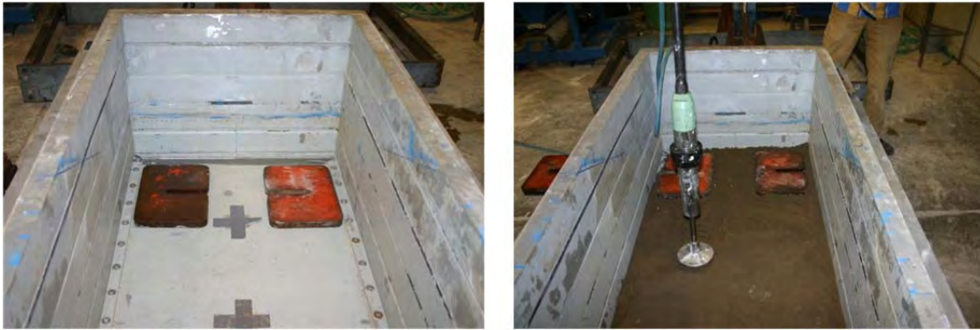
Figure 8.7 Construction of asymmetric model GC03 with counter weights placed inside the container.
