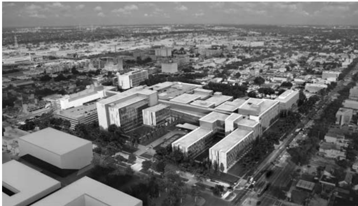
FIGURE 5.6 New Orleans Downtown Hospital Complex.
