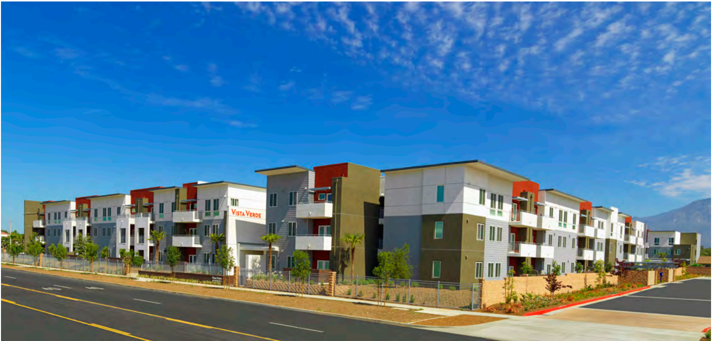
Completed construction of the Vista Verde Apartments. Photo credit: National Community Renaissance
