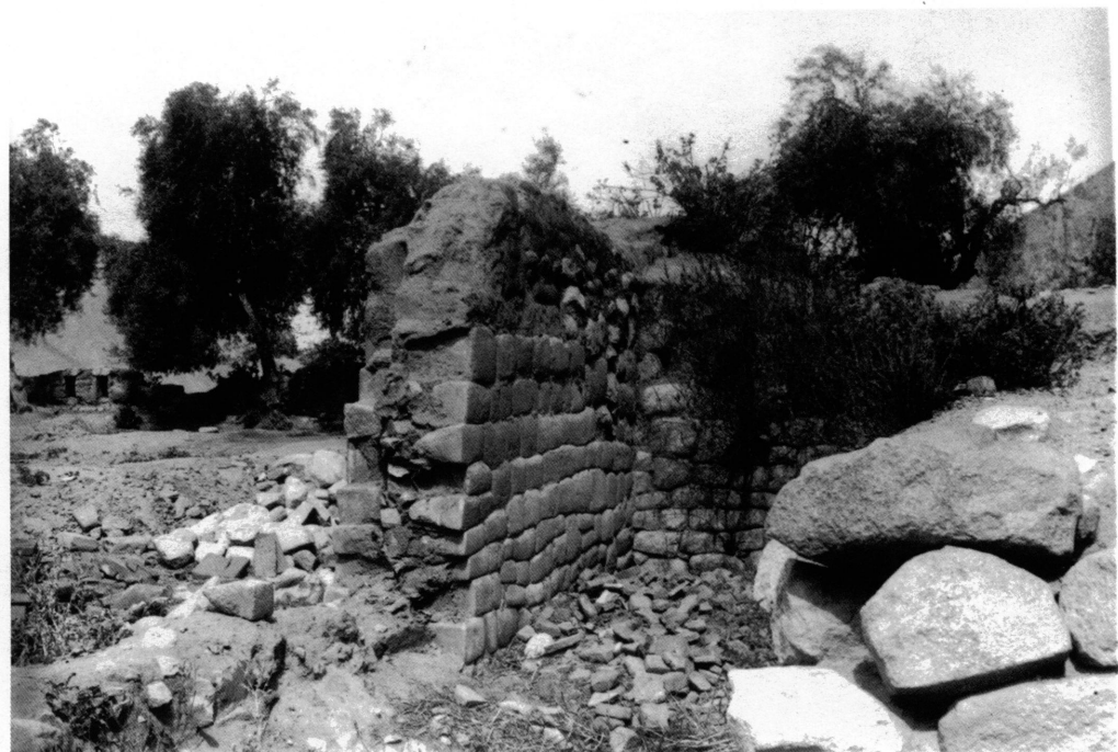
No. 1275 Wall construction with wedge stones (Huaytará)
