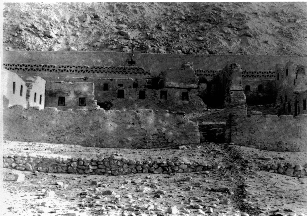
No. 1164 View from U1 towards N on axis (TC)
