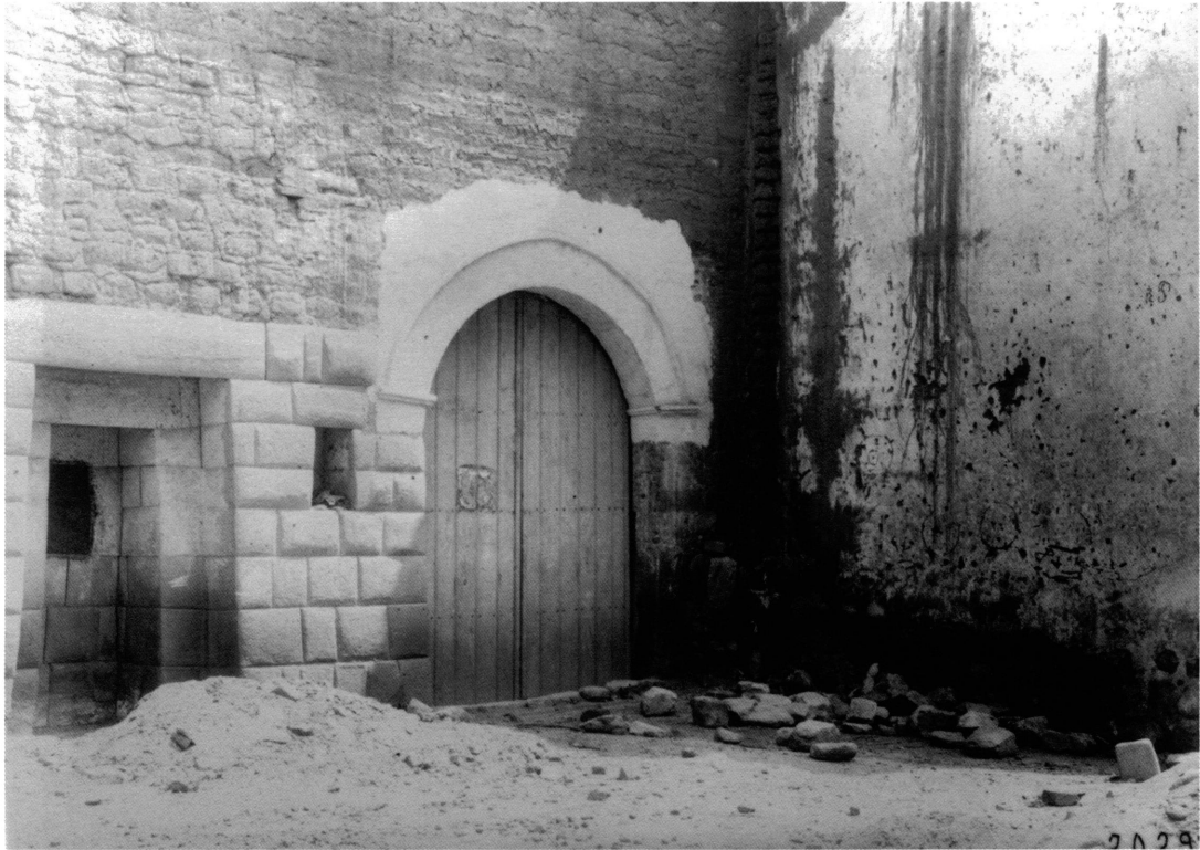
No. 1278 S façade of church, eastern most niche with modern archway (Huaytará)
