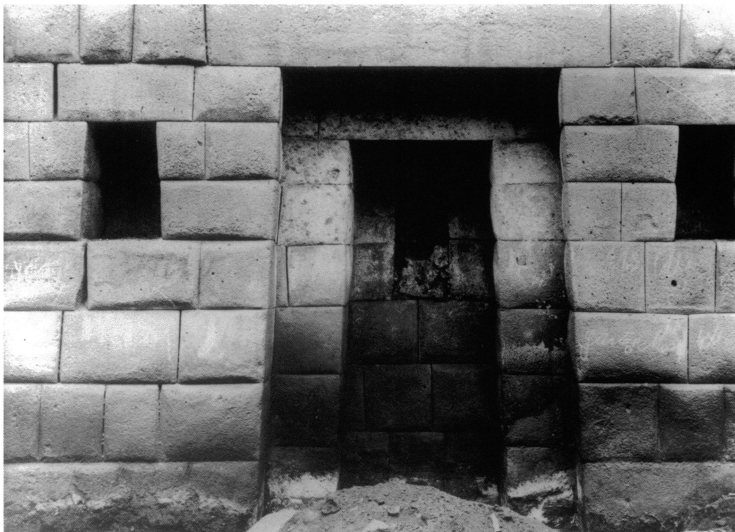
No. 1305 Church, S façade, niche 2 (counting from E), example of ashlar masonry (Huaytará)
