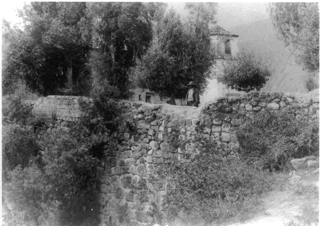
No. 1302 Western retaining wall of churchyard (Huaytará)
