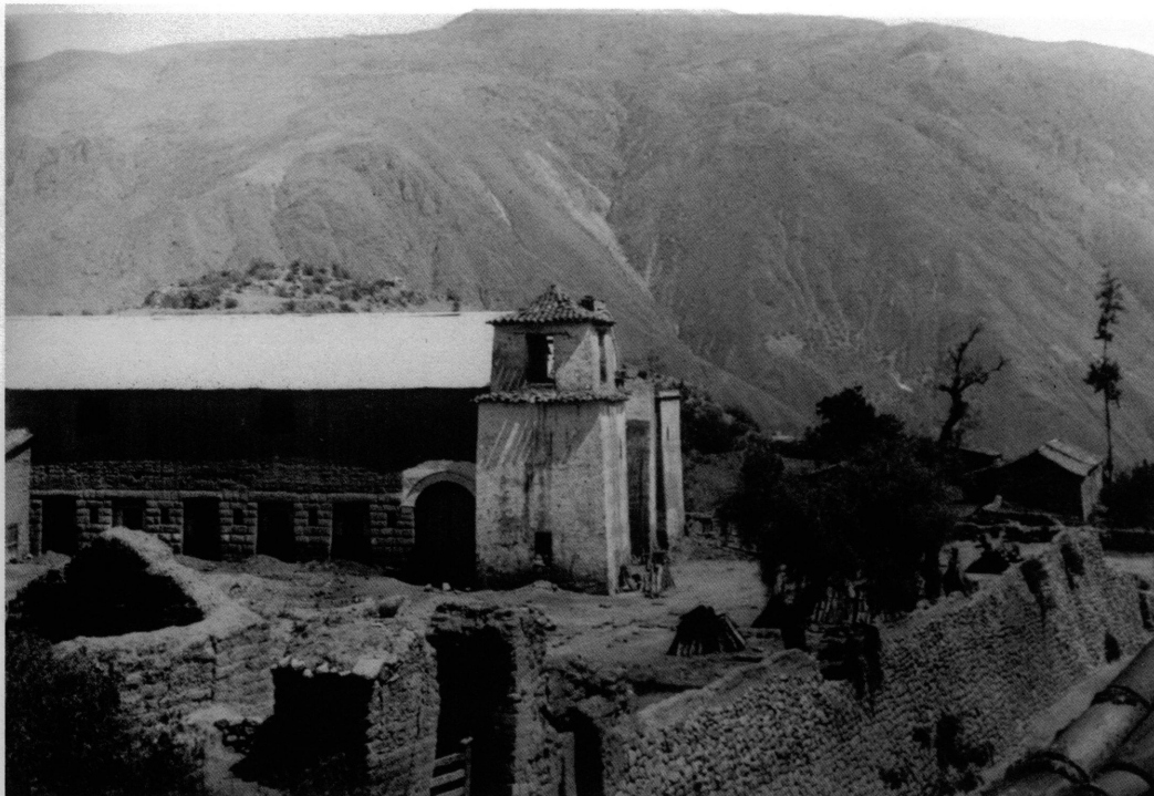
No. 1272 Church, churchyard, retaining wall on east side, seen from south (Huaytará)
