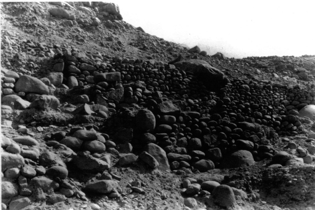
No. 1190 Terraces with drain (river cobble construction), left bank opposite TC
