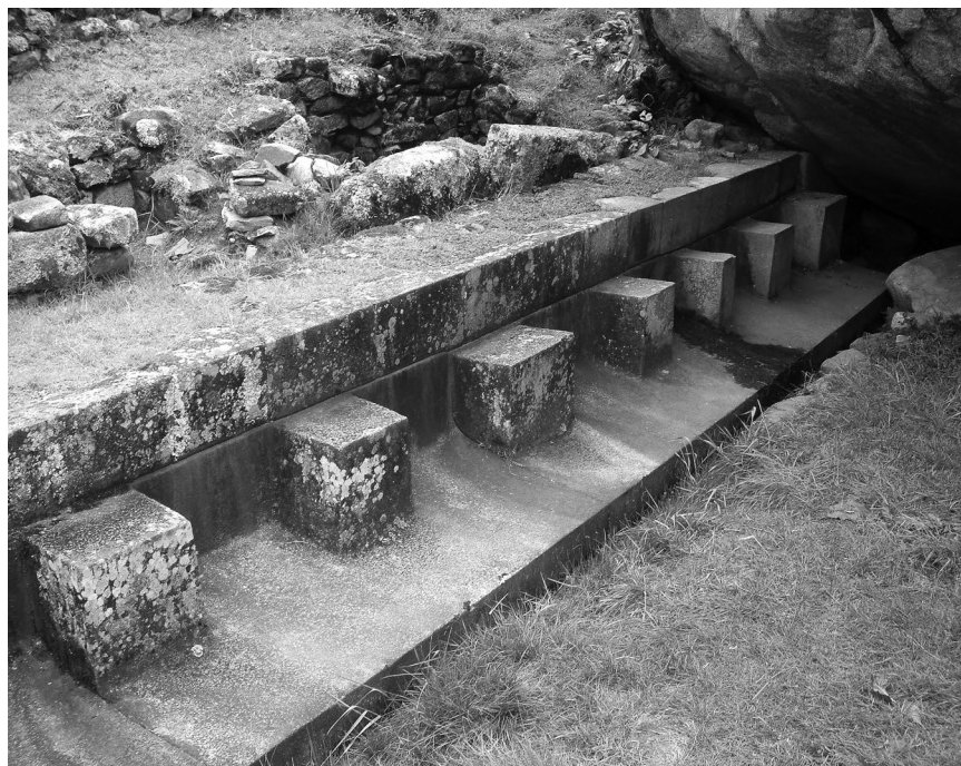
Figure 3.18. A finely carved bench at the base of Yurak Rumi marks the emergence of a sacred spring (photograph by Brian S. Bauer and Miriam Aráoz Silva).
