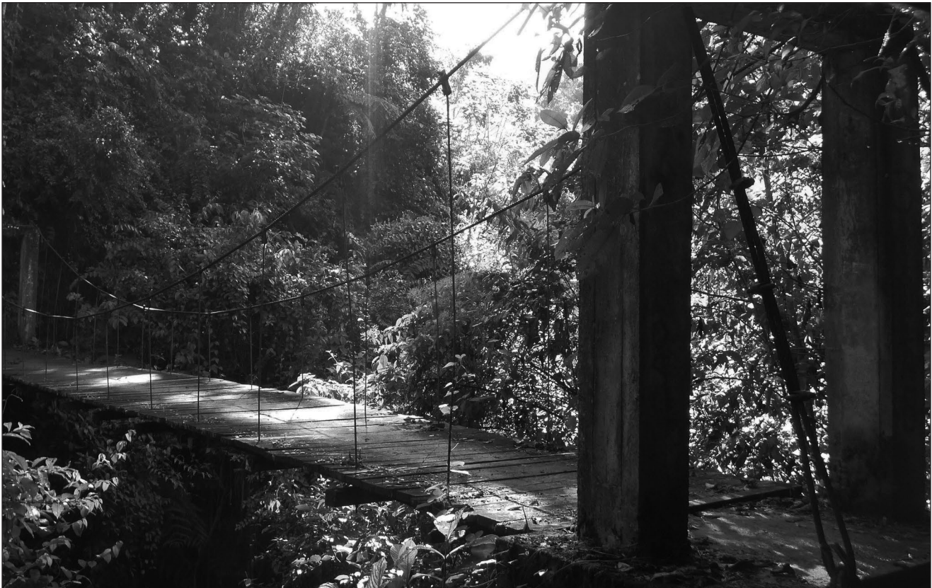
Figure P.1. The last of three suspension bridges built between Azulmayo and Espíritu Pampa, 2010 (photograph by Brian S. Bauer and Miriam Araújo Silva).
