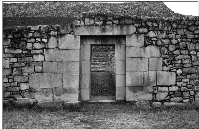
Figure 1.11. Doorway at Vitcos (Rosaspata) after reconstruction (photograph by Brian S. Bauer and Miriam Aráoz Silva).
