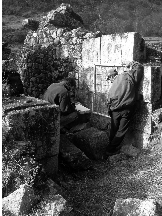
Figure 3.28. (left) The large passageway stone blocks at Yurak Rumi (photograph by Brian S. Bauer and Miriam Aráoz Silva).
