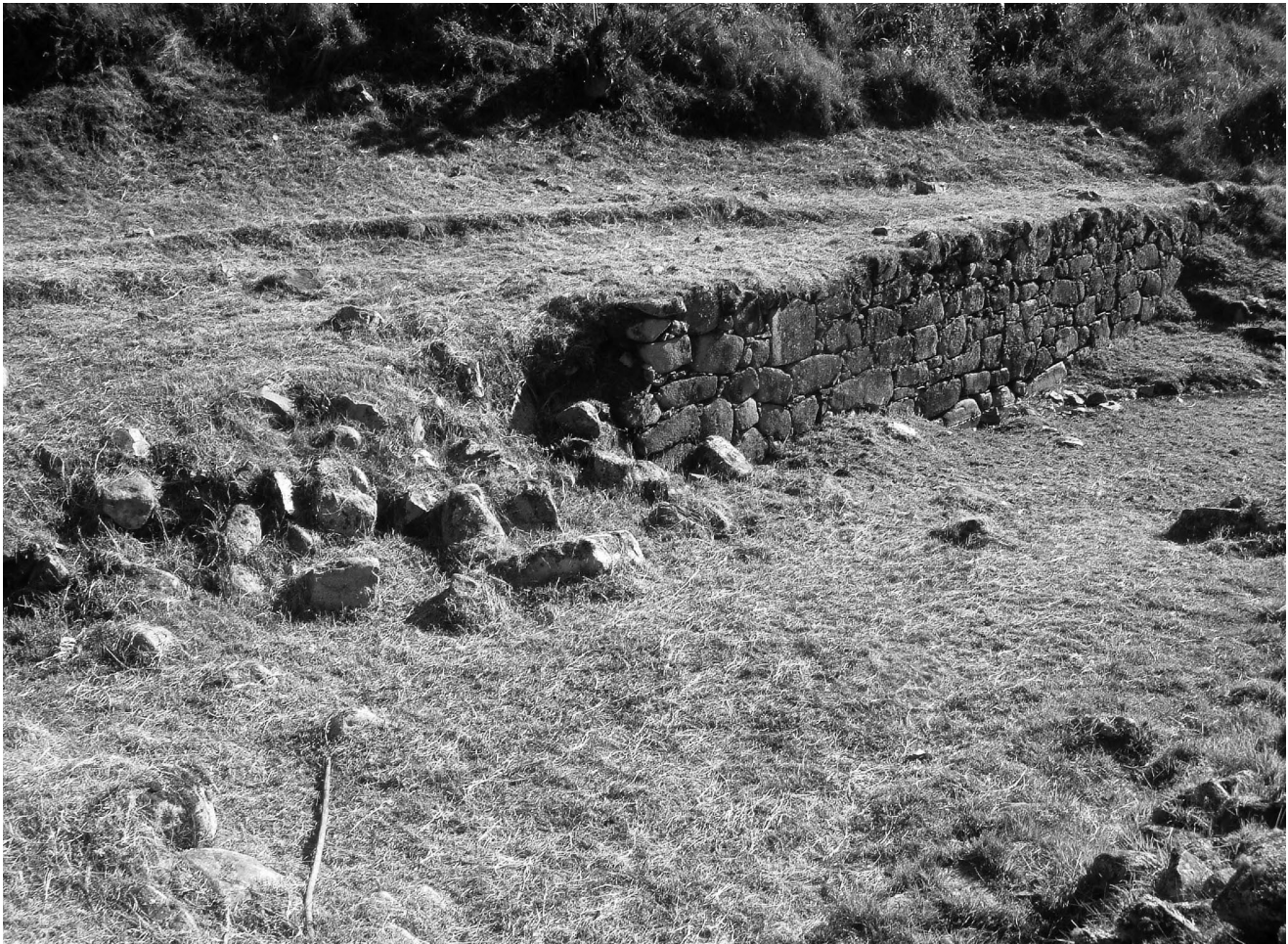
Figure 3.31. The third and lowest terrace of Yurak Rumi is made with large, well-worked stones (photograph by Brian S. Bauer and Miriam Araújo Silva).
