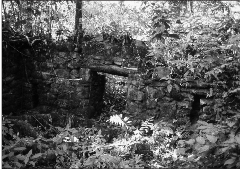
Figure 5.18. Building 5 in 1983. Parts of the gable can still be seen above the doorway (photograph by David Drew).
