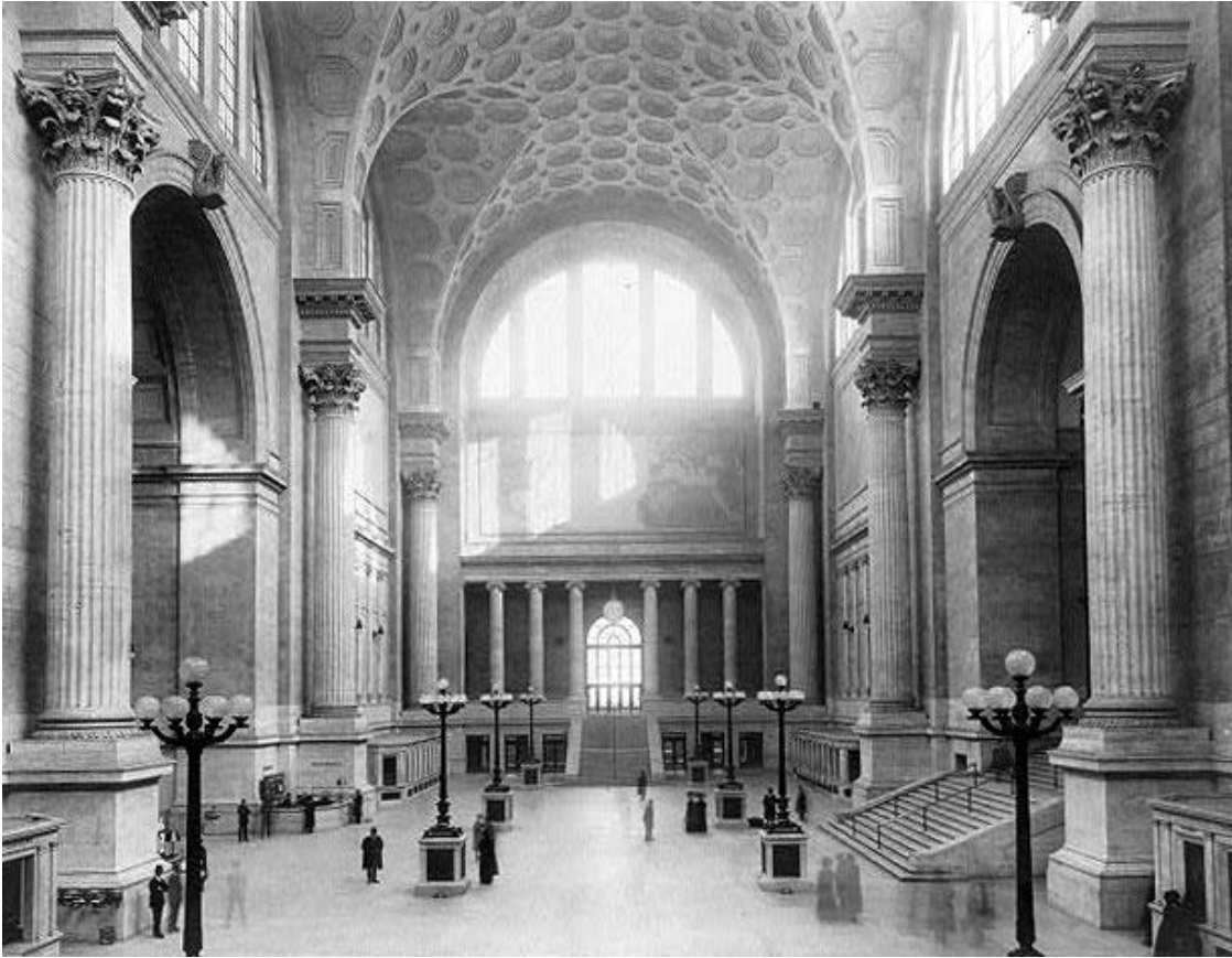
Figure 30. Main waiting room, Pennsylvania Station, ca. 1911.
