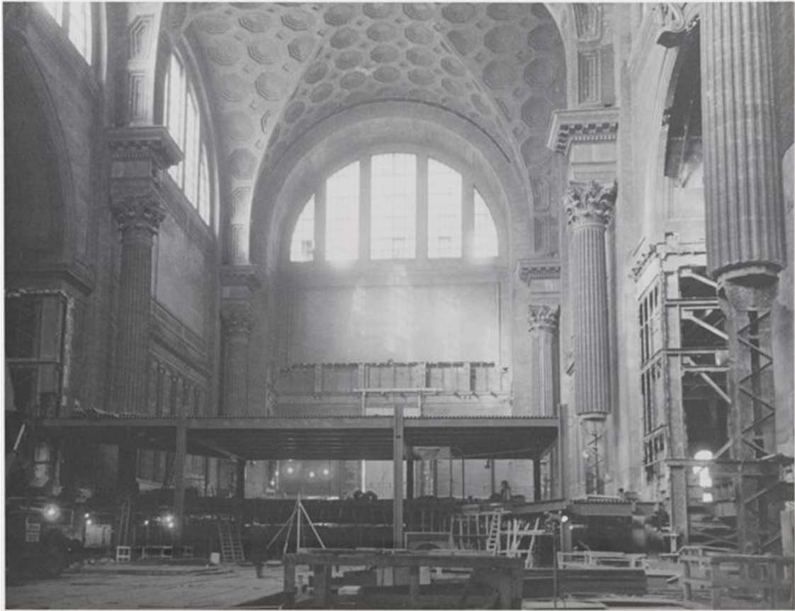
Figure 36. Interior Demolition of Pennsylvania Station, 1964-1965.
