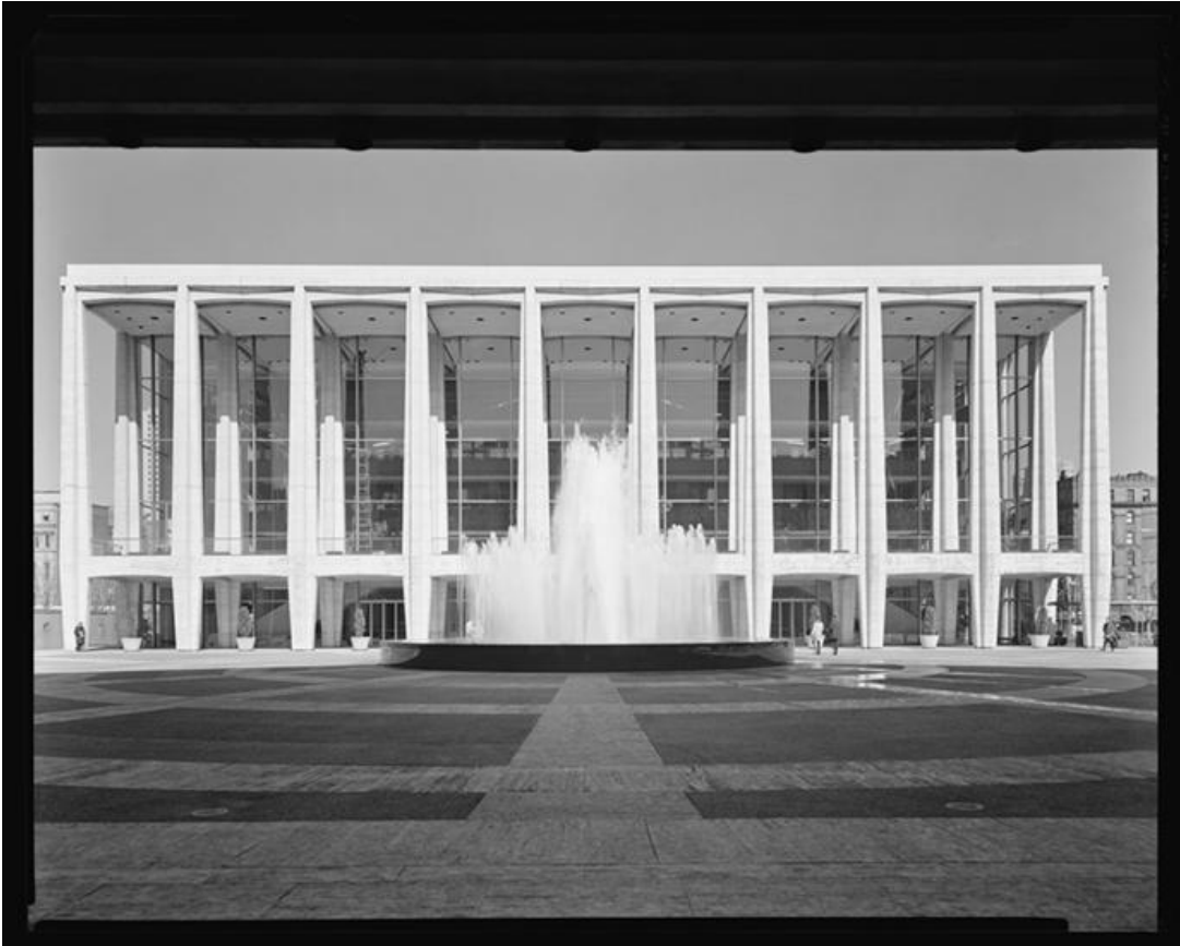
Figure 23. Philharmonic Hall (now Avery Fisher Hall), front elevation, Lincoln Center, New York, NY, 1965.
