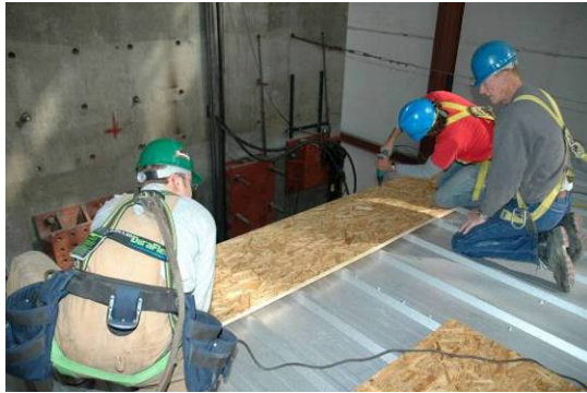
Wood Panel Screwing
