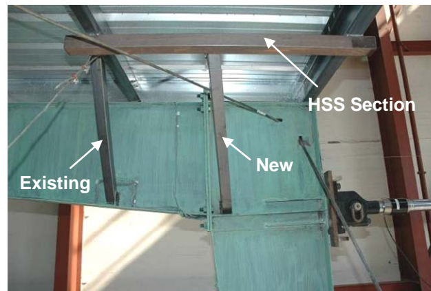
(b) Additional Flange Brace on South Side of Frame 2
