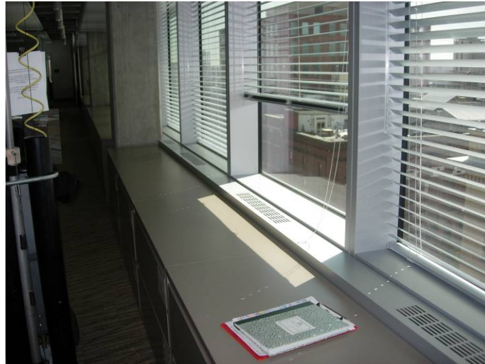
Figure 4: Typical perimeter sill diffusers for UFAD floors
