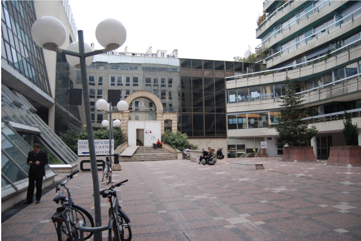
Figure 5. Courtyard of old Baccarat factory at 30 bis rue de Paradis. Note the nineteenth-century entrance and staircase in the center of the photograph, the only part of the original structure that was kept. (Author's photograph, April 7, 2010)
