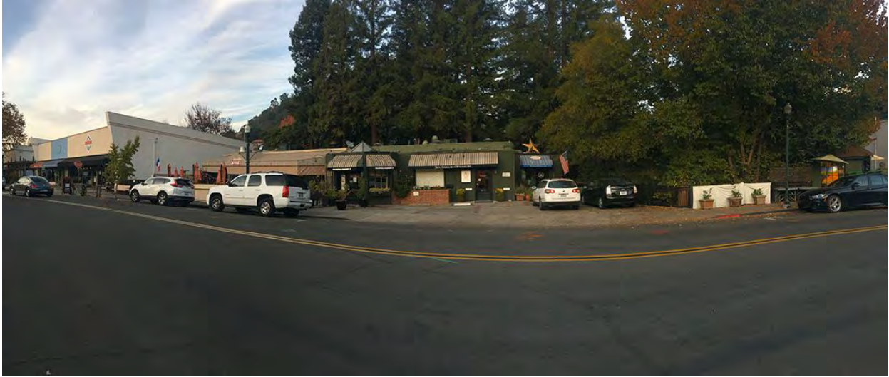
(Fig 23. Front view of structures to be taken down)
