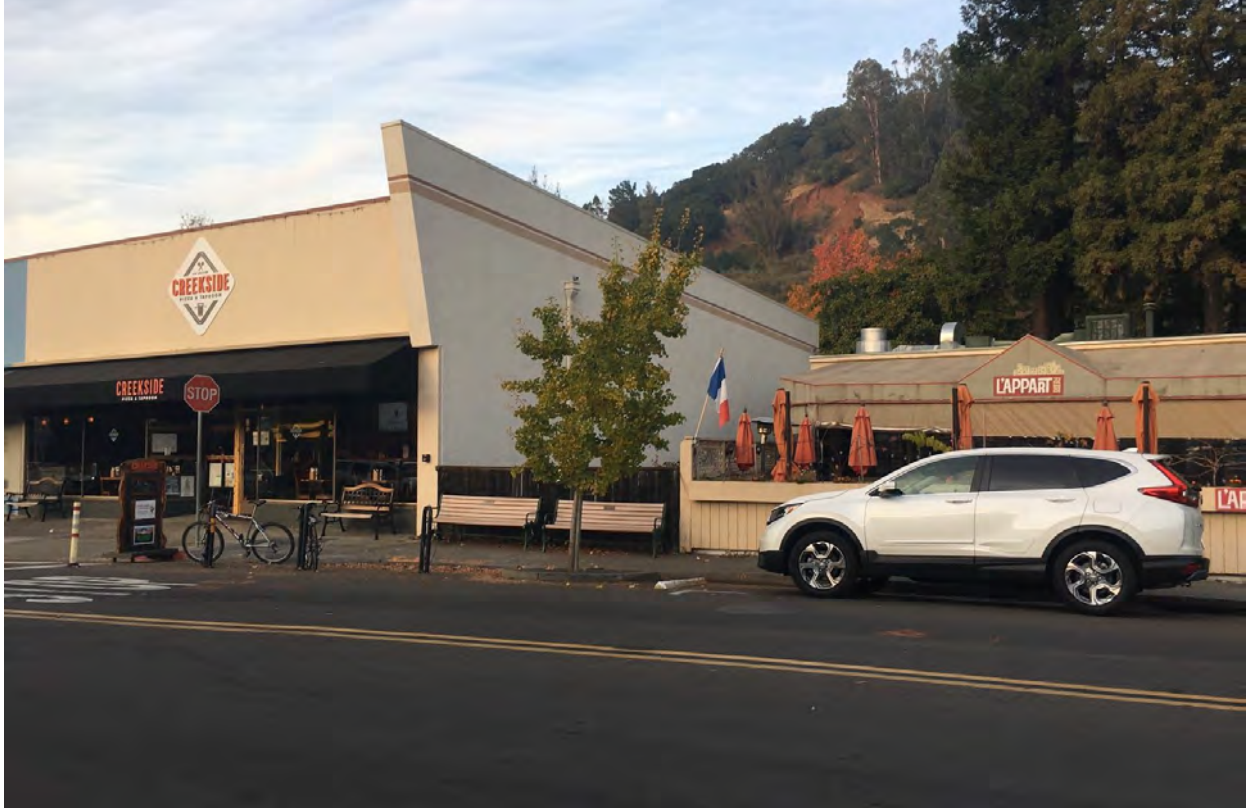
(Fig 31. Front view of Creekside Pizza and the Lappart business that will be demolished for visual improvement, labeled D in Fig)
