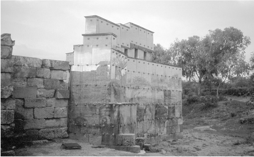
FIGURE 18.2. Protective panels of Perspex/Plexiglas bolted to the ancient mud brick walls at Gela city-state, 1984. Note the development of plant growth between the panel and wall surfaces.
