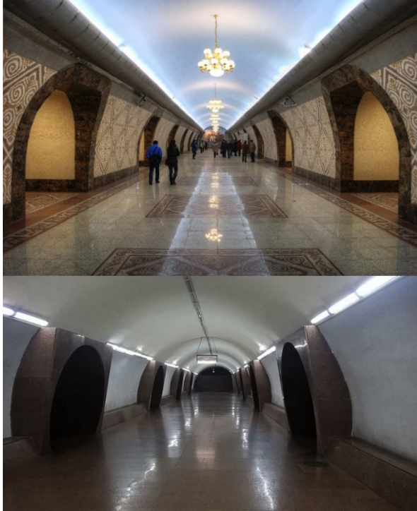
Figure 4. Above: Almaty Station in Almaty. Below: General Andranik Station in Yerevan. Both are deep pylon stations.
