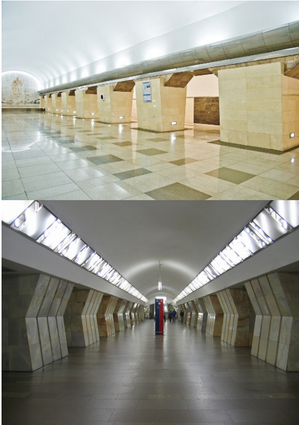
Figure 5. Above: Abay Station in Almaty. Below: Sukharevskaya station in Moscow. Both are deep column stations.
