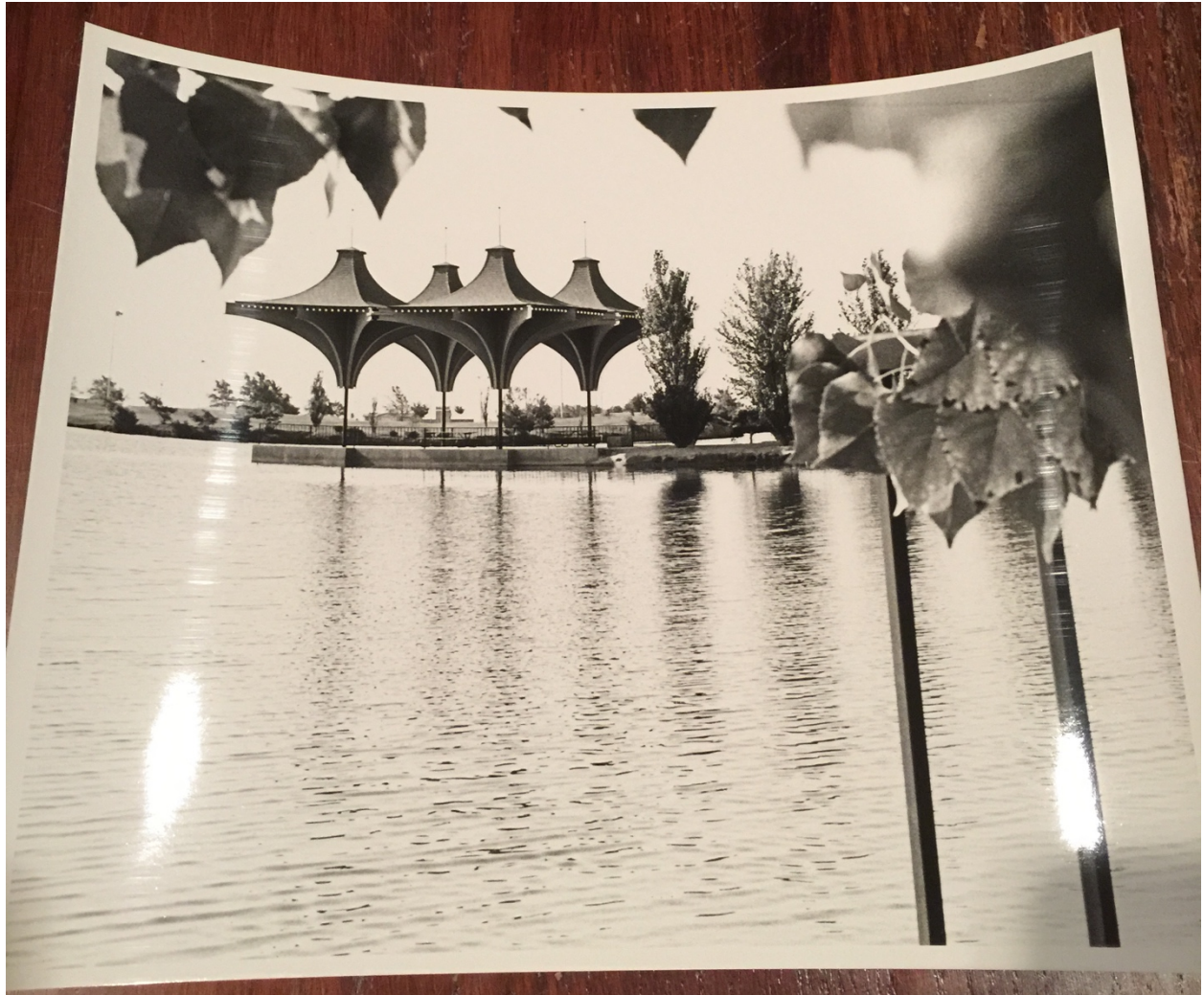
Figure 1.24: Smith and Williams, Architects and Engineers, Central Lake Pavilion, California City , Date Unknown. Photograph by Venturi and Rauch, Architects and Planners. Courtesy The Architectural Archives, University of Pennsylvania by the gift of Robert Venturi and Denise Scott Brown.
