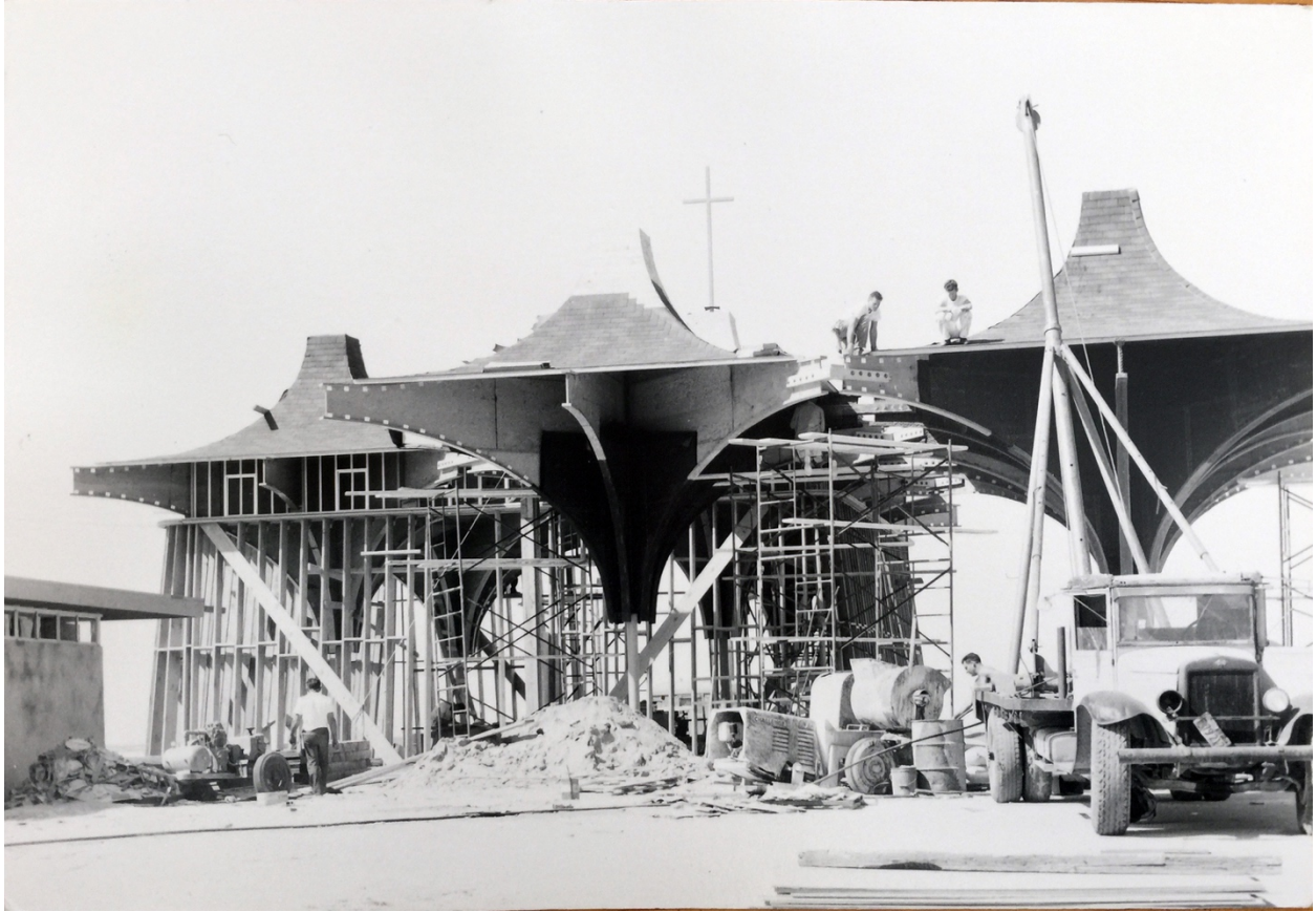
Figure 1.23: Smith and Williams, Architects and Engineers, Congregational Church, California City , 1961. Courtesy Architecture and Design Collection, Art, Design & Architecture Museum, University of California, Santa Barbara, CA.
