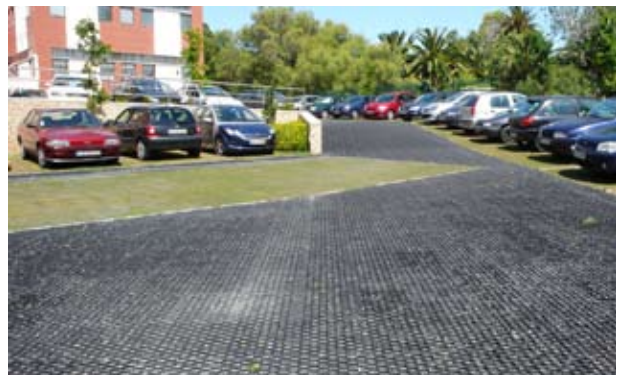
Pervious paving in a parking area in Cascais includes both planted and gravel. Cobblestone paving can also be pervious when the sand is not heavily compacted.
