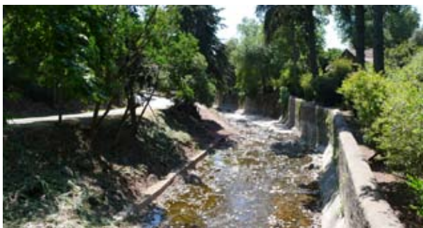
Ribeira da Barcarena channelized conditions
