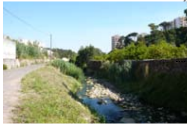
Existing Abandoned Road
