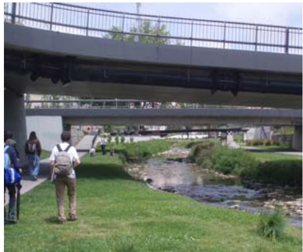
Walking underneath a roadway bridge at the Cacem Polis project.
