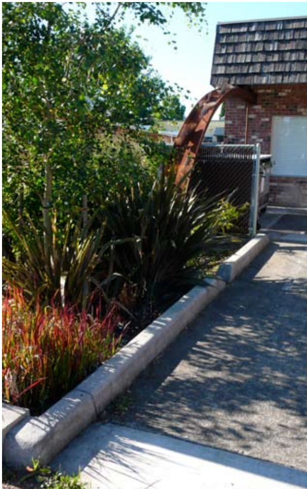
A raingarden in Portland, Oregon accepts runoff from the roof of the adjacent building.
