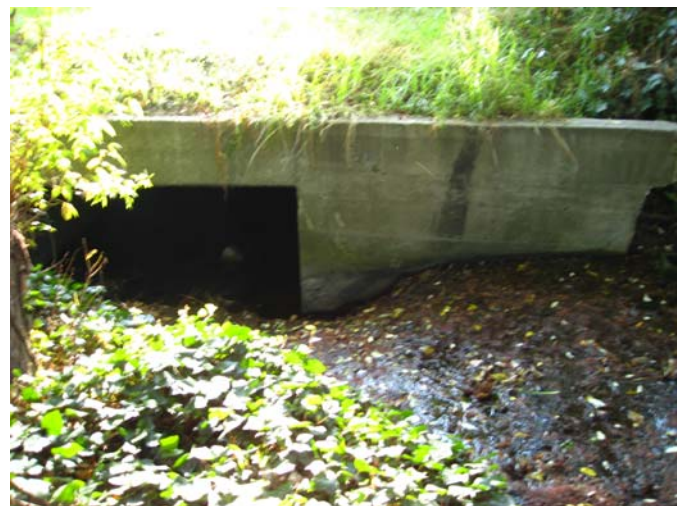
Figure 7: Codornices Creek entering the 10th Street Culvert.
