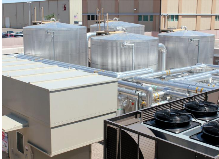
Figure 33: Natural gas generator at the Aperture Center microgrid
