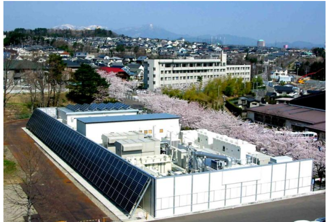
Figure 4: Overhead view of the Sendai energy center
