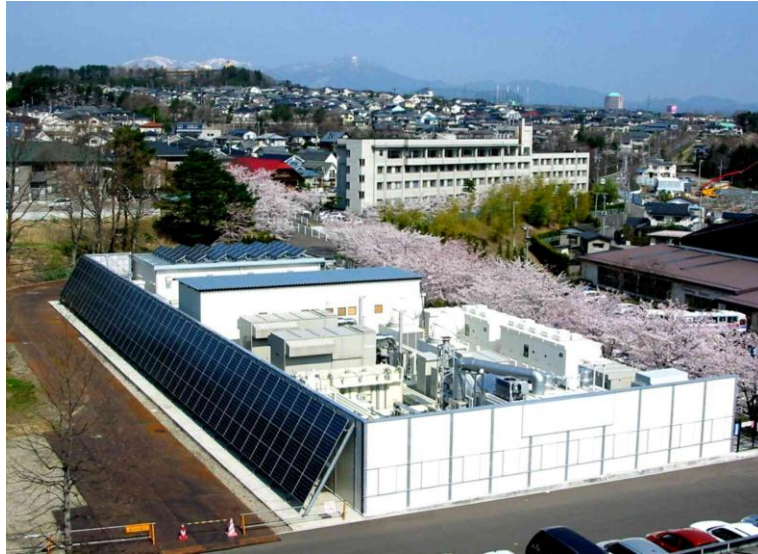
Figure 18: Overhead view of the Sendai energy center
