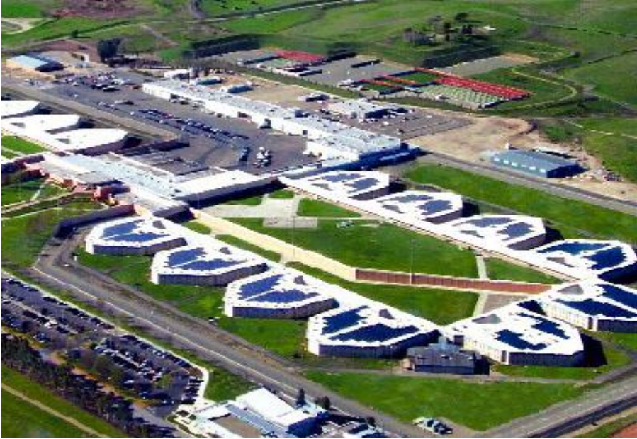
Figure 16: Overhead view of the Santa Rita Jail showing the rooftop PV array
