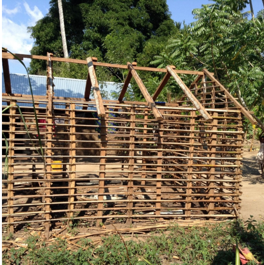
Figure 16-8. House frame, with thatch before earth is applied.
