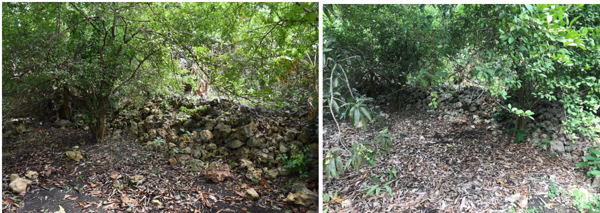
Figure 8-10. Stone walls at base of path leading down plateau.
