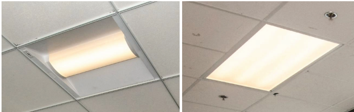
Figure 10. Luminaires used in the tests: LED luminaire ( left ) and fluorescent troffer ( right ).
