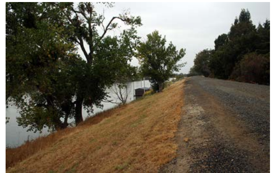
Figure 25: The image of levee
