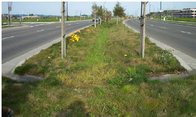
Figure 76-77: The images of street bioretention planters at the street median
