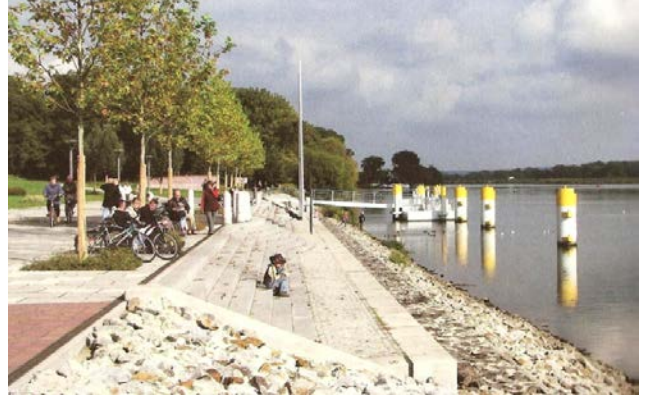
Figure 61: The image of the seating steps at the canal-faced side of section C-2
