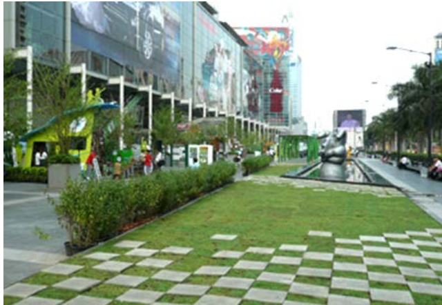
Figure 64: The image of disconnected impervious areas and using pervious pavement for plaza
