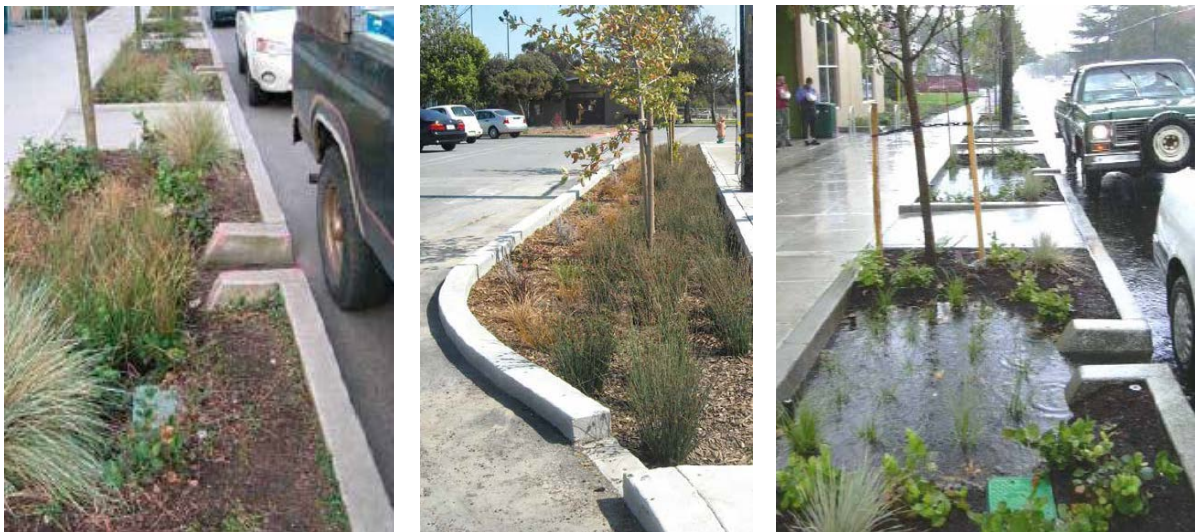
Figure 82-84: The images of street bioretention planters at the sidewalks
