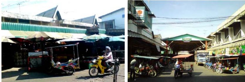
Figure 43-44: Existing market building
