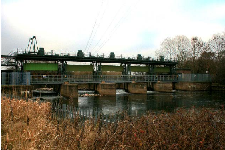
Figure 30: The image of sluices and pumping station
