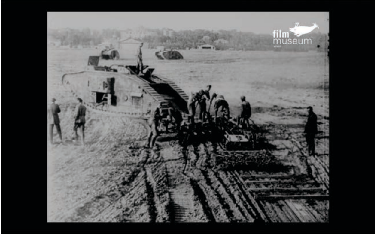
FIGURE 3.8. Tanks repurposed as tractors leveling an airfield. From Dziga Vertov, Kino-Pravda , no. 7, 1922.
