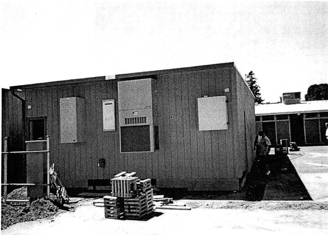
Figure 3: Photograph of the back walls of joining modules for a HPCBS Element 6 RC, each with mounted components of the standard or IDEC HVAC system.
