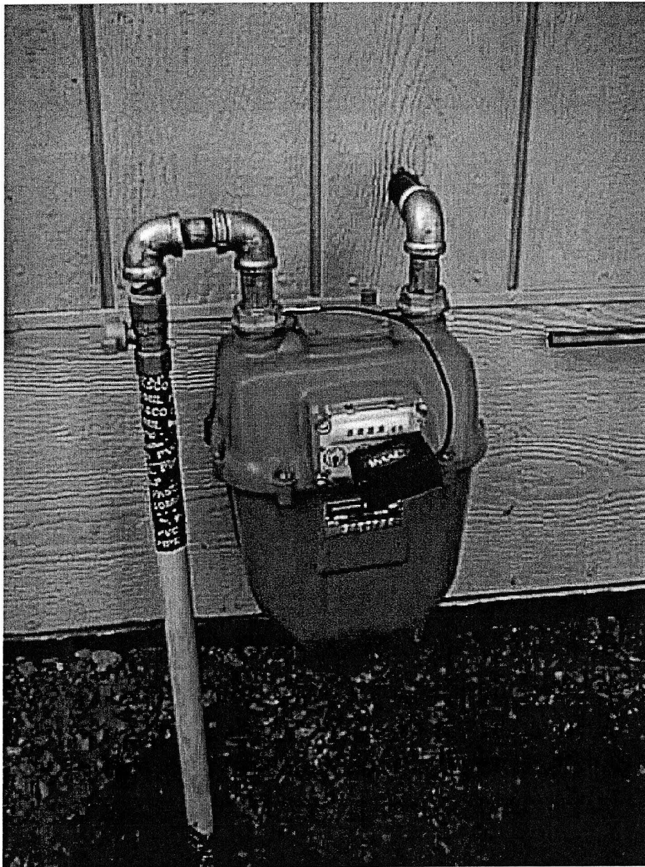
Figure 11: Photograph of the advanced HVAC system's water heater gas usage sensor (Equimeter 275P) for the energy monitoring component of the field study.
