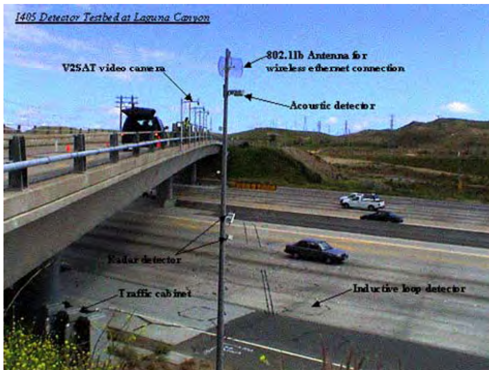
Figure 5.1 Upstream of TDS 2 on Northbound I-405 freeway (Laguna Canyon)
