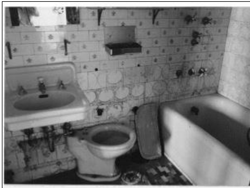
Figure 92: Mission Inn bathroom before renovation. Photo courtesy Mission Inn Foundation & Museum.
