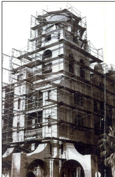
Figure 96: Scaffolding encompassing the Cloister Wing. Photo courtesy Mission Inn Foundation & Museum.
