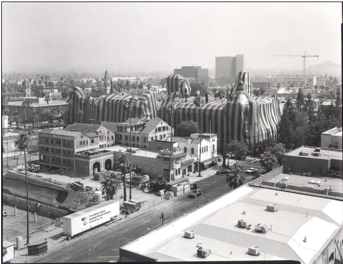
Figure 94: Due to the Mission Inn's termite infestation the entire hotel had to be tented for termites in 1987. Photo courtesy Mission Inn Foundation & Museum.
