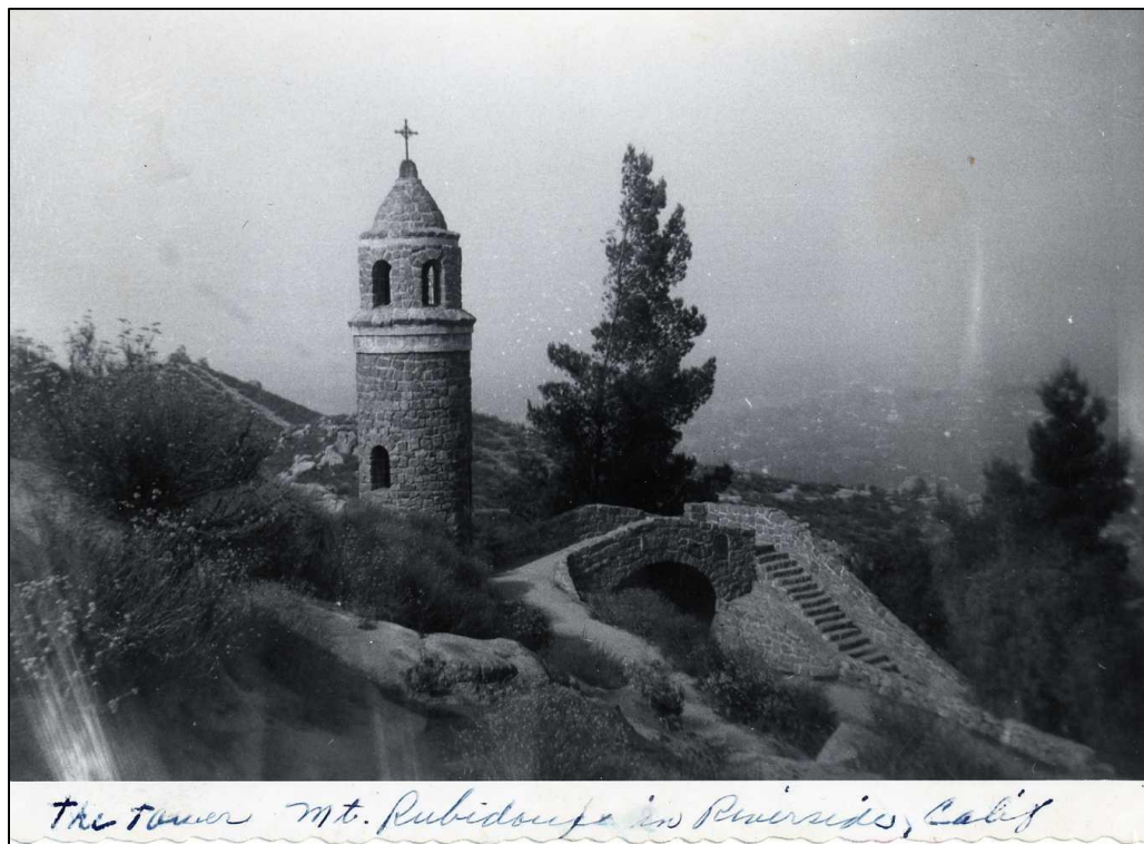
Figure 62: The Arthur Benton-designed Peace Tower at Mt. Rubidoux dedicated to Frank Miller in 1925. Photo courtesy Riverside Metropolitan Museum.
