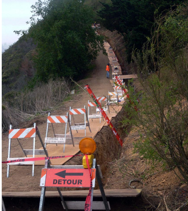
Figure 4-53. View of TR-4 [TR4?] along Panoramic Road
