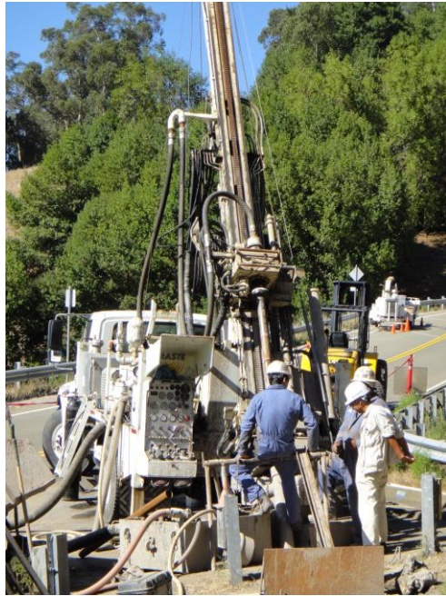
Figure 3-5. Drilling of WF-5. Note that it is a 60° inclined drilling.
