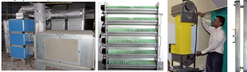
(6) Dedicated Outdoor Air System and direct evaporative cooling of fresh air using exhaust air (left), with various components and sub-systems (right)
