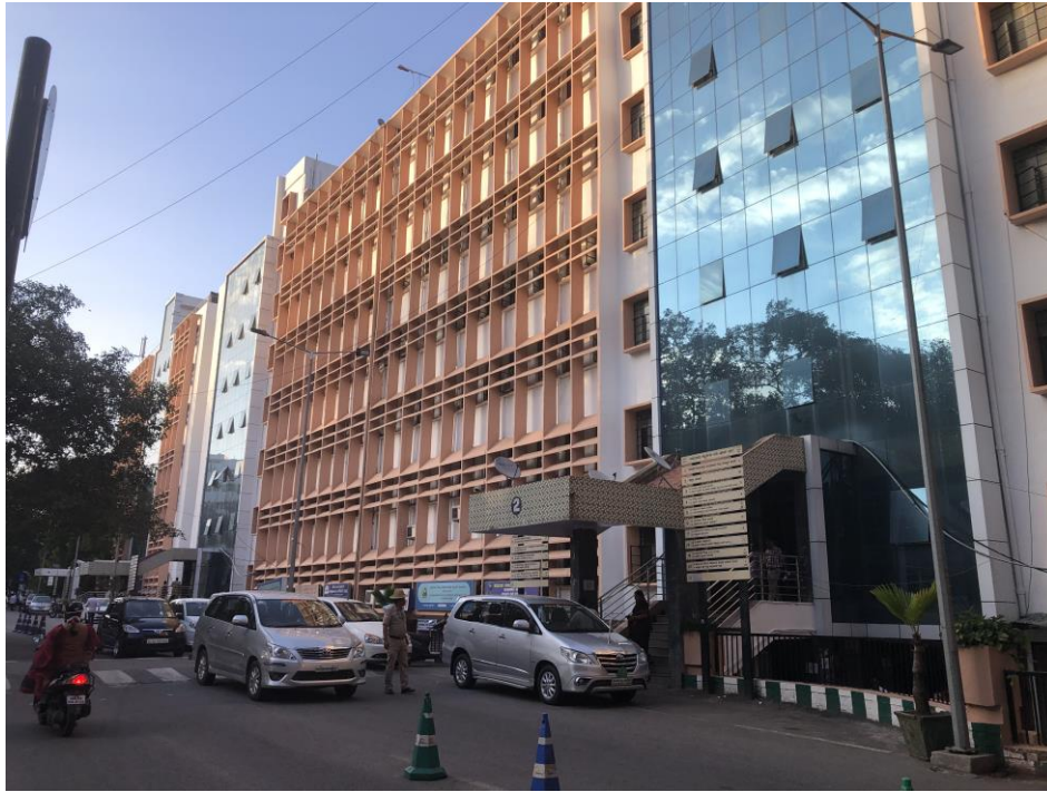
Figure 2: Typical facades of commercial buildings in India, showing the changing trends from thermally massive construction with punched windows to fully-glazed facades.
