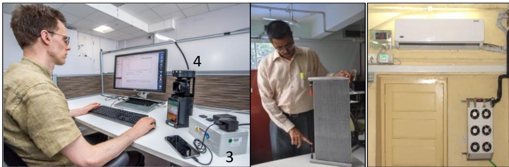
(3) Smart Strip, and (4) SPACE Smart Hub for workstations (left), (5) Novel microchannel heat exchanger design of the 5 TR Split unit
