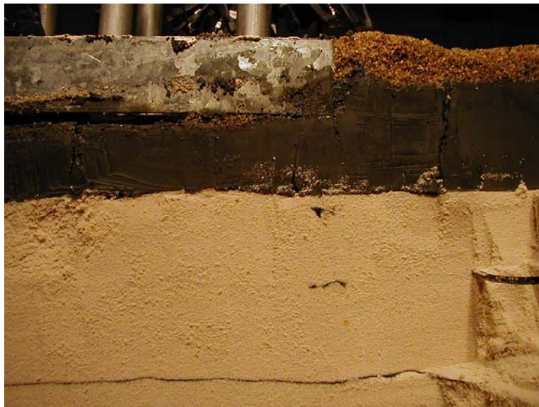
Figure 6. Side view of the piles beneath the cap after the adjacent soil has been excavated (Note the sand that has boiled into the gaps behind the piles, as the clay spread from right to left).
